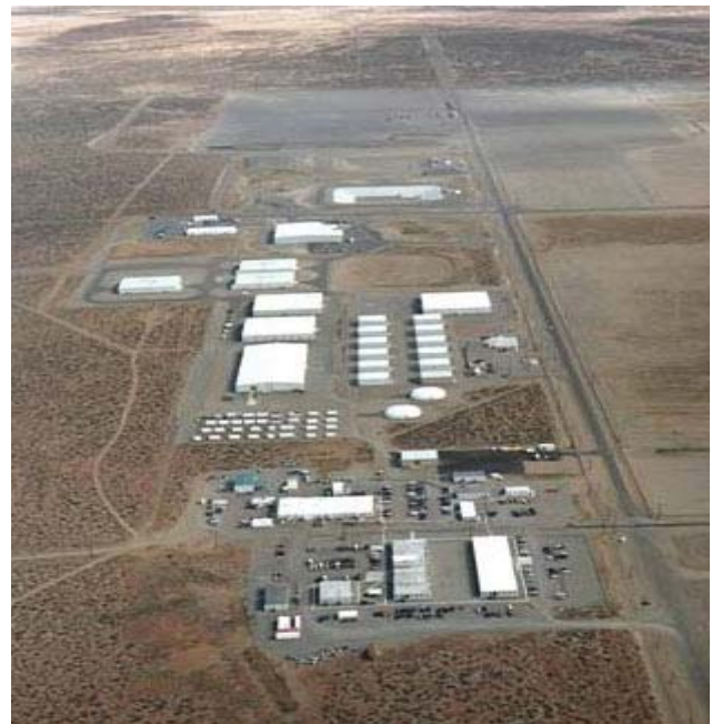
Solid Waste Storage and Disposal Facilities
