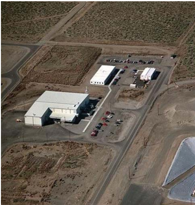
Waste Receiving and Processing Facility
