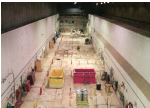
T-Plant Canyon Deck
