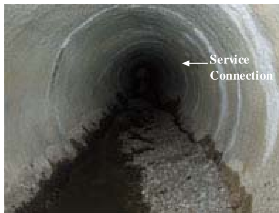
Gravel Deposit Upstream of Meter Pit
