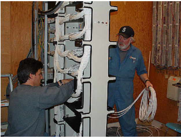
New LAN Installation
