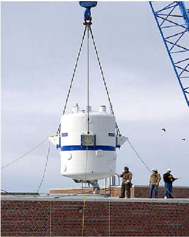
Installation of 16-ton Superconducting Magnet at EMSL
