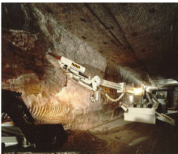
Scaler Miner Removing Loose Rock in the WIPP Underground
