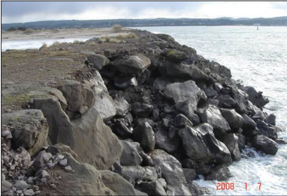
Figure 6. Repair Area 2, Seaward Scalloped Area at Stations 62+00 to 64+00
