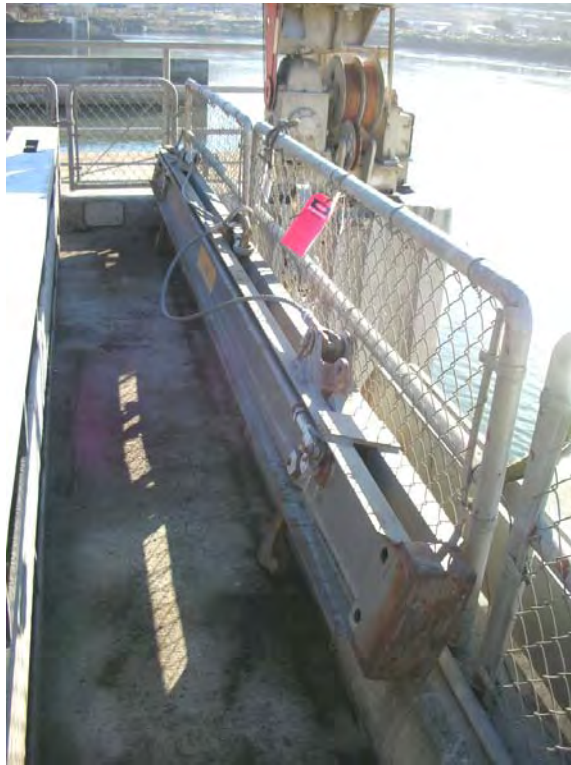
M-4 Entrance Weir Lifting Beam
