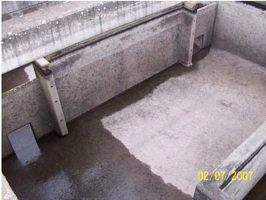
Photo H-11 Typical East Ladder Weir
