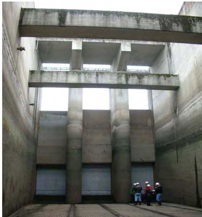
Photo ME-5 Water leaking past downstream bulkhead in collection channel
