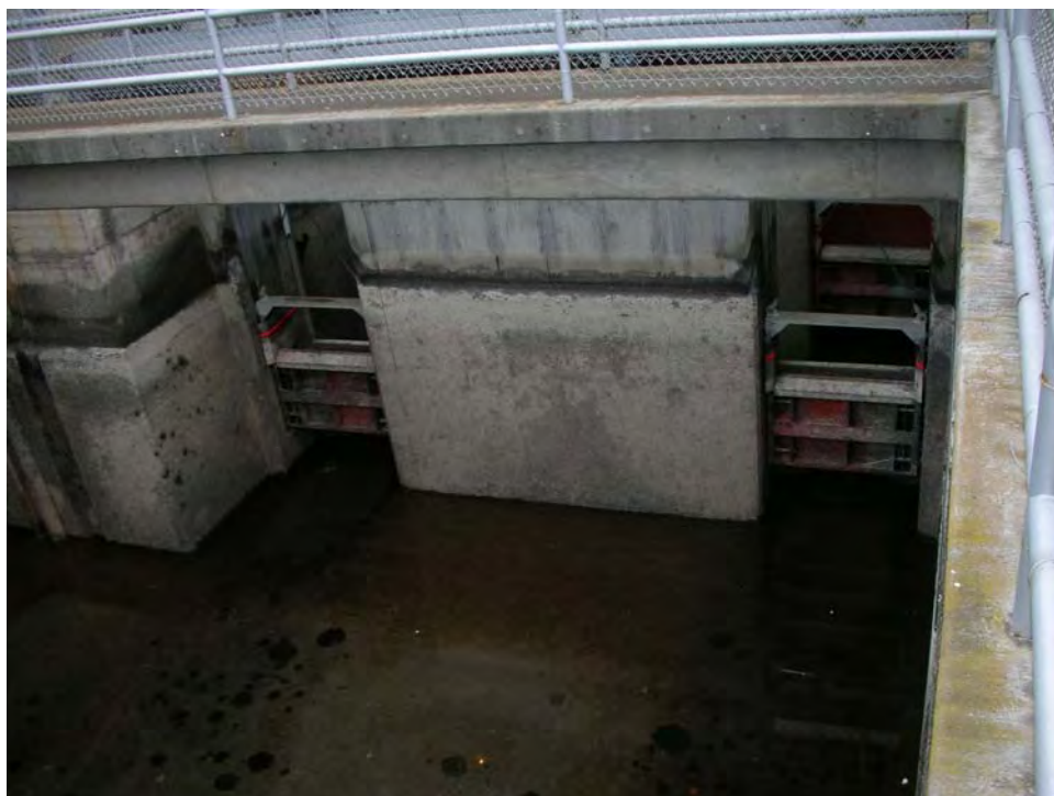
Photo ME-20 Weirs fabricated from a former single weir
