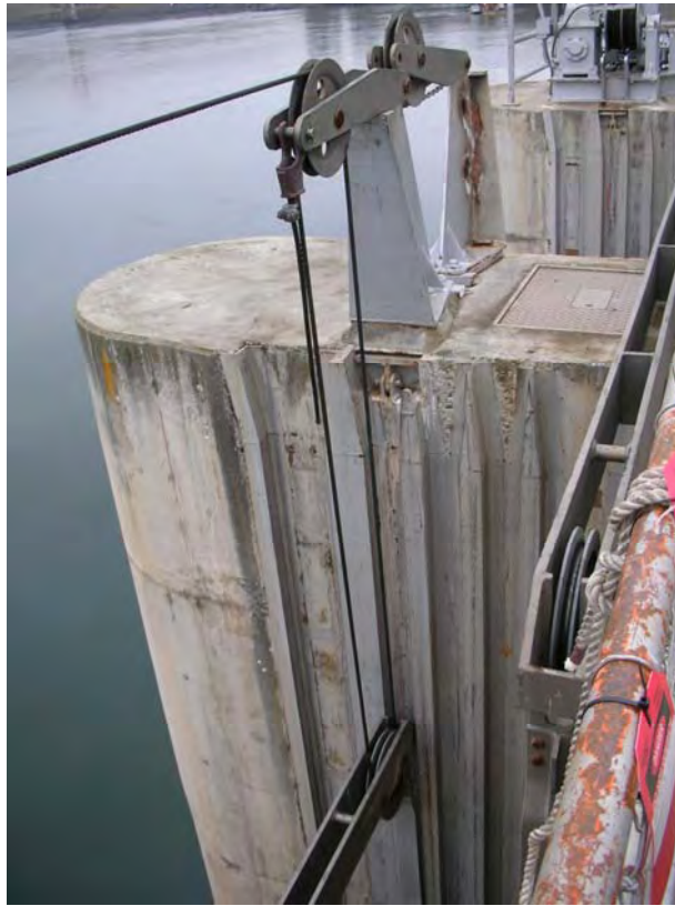
Photo ME-9 Dual sheaved lifting beam for raising and lowering telescoping weirs
