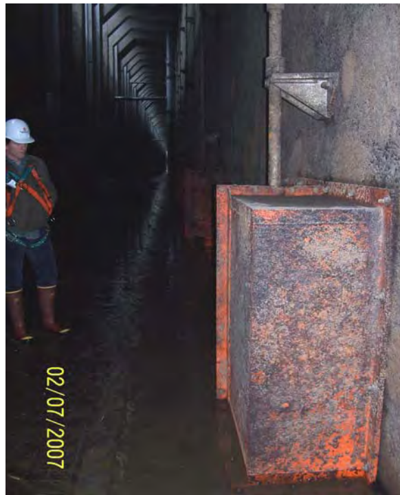
Photo H-6 Diffuser Gate Housing
