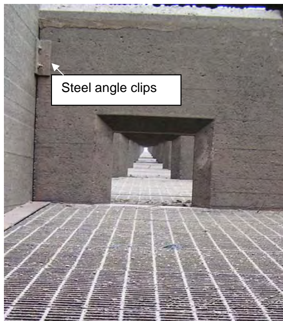
Photo CS-4 – East Fish Ladder Concrete Weir supported by steel angle clips
