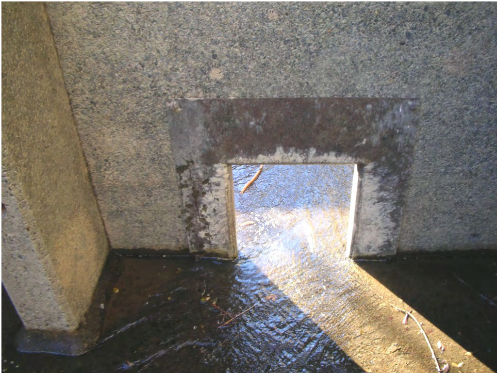
H-14 Modified Orifice
