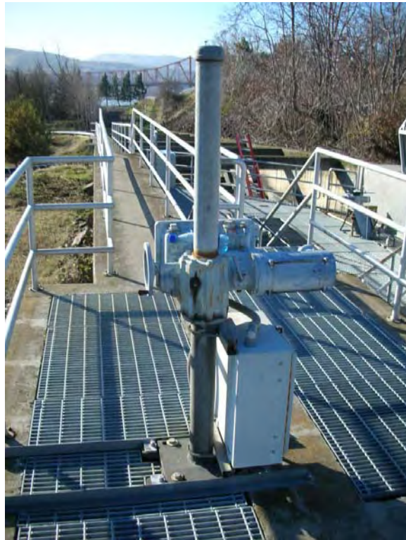
M-12 Juvenile Fish Bypass Gate Actuator
