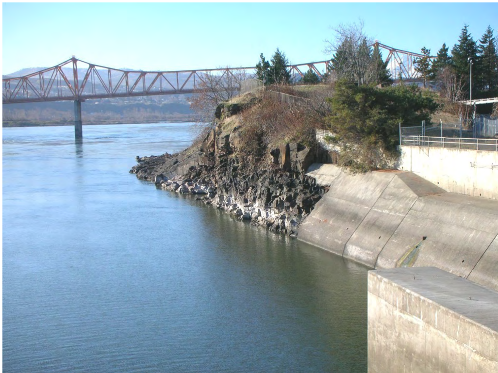
G-2 North Shore View Looking Downstream
