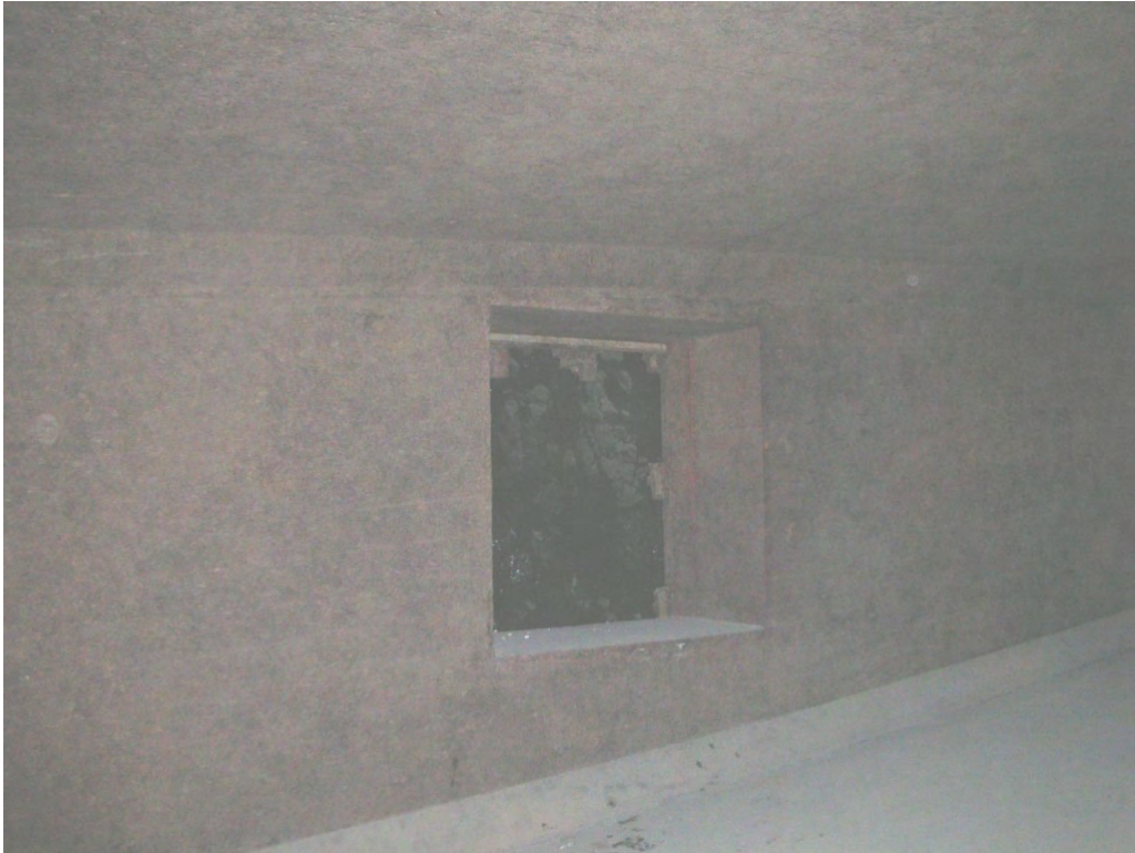
H-1 Diffuser Gate
