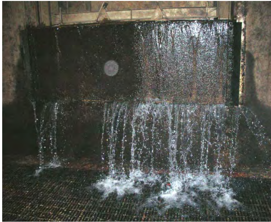
Photo ME-5 Water leaking past downstream bulkhead in collection channel
