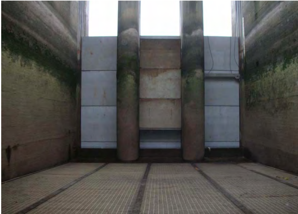
Photo ME-1 Bulkheads present in the three east fish entrance gate openings
