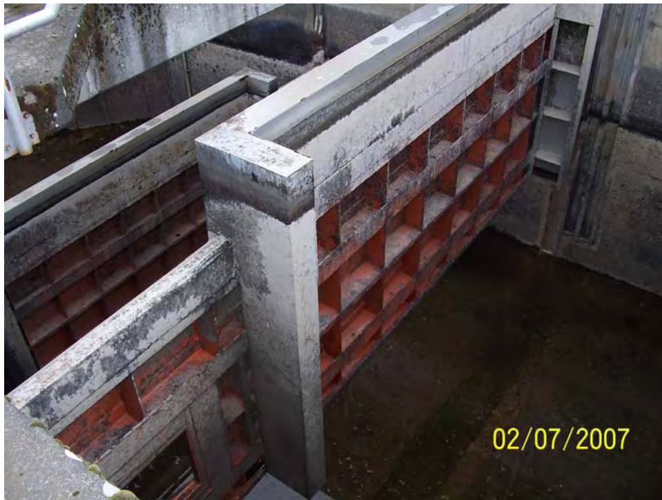
Photo H-13 Exit Section
