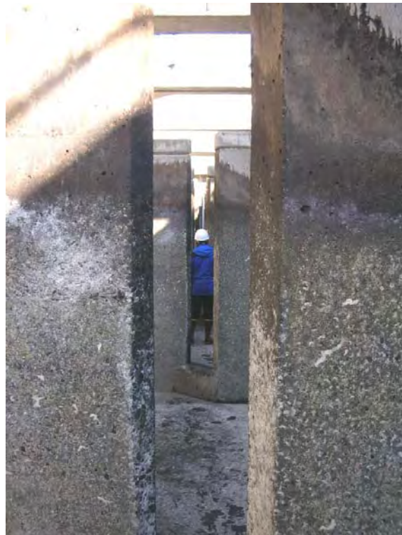
H-10 Vertical Weir Slot Looking Upstream
