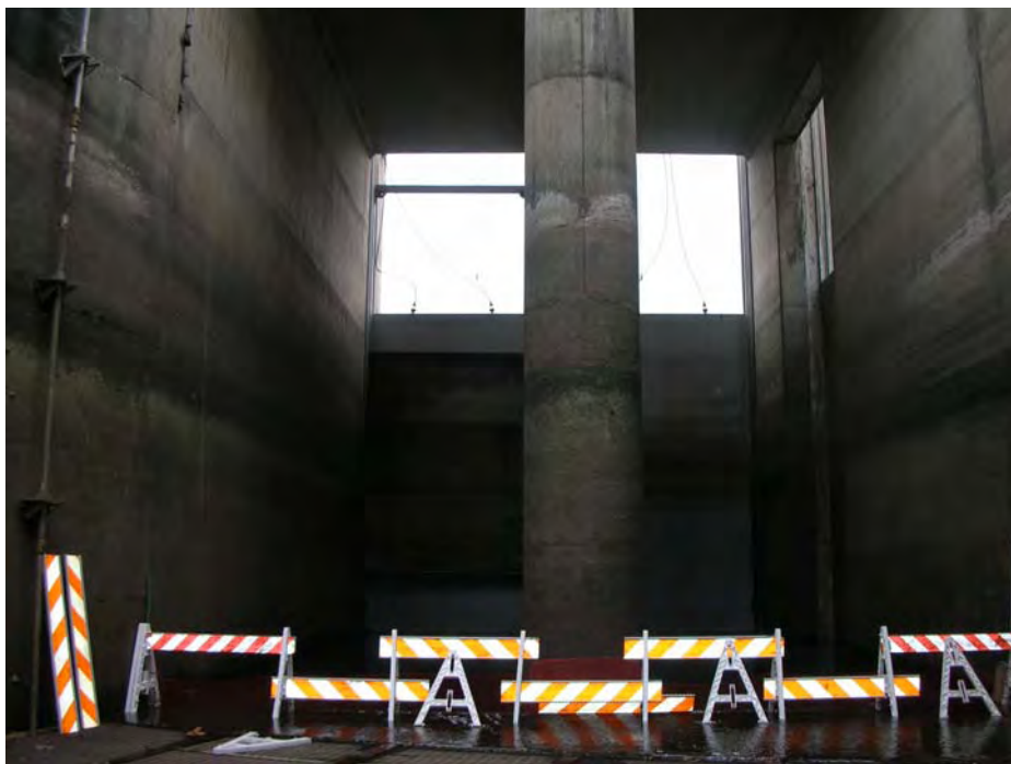
Photo ME-8 South fish entrance bulkheads
