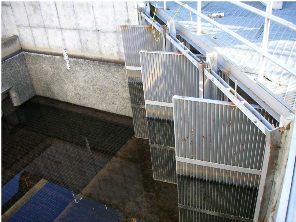
H-12 Counting Station Floor Diffuser Grate and Picket Leads
