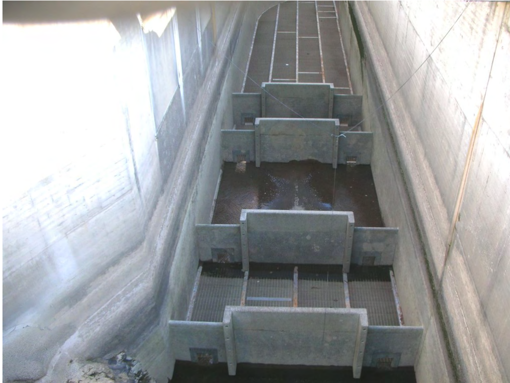
H-7 Floor Diffusers and Weirs
