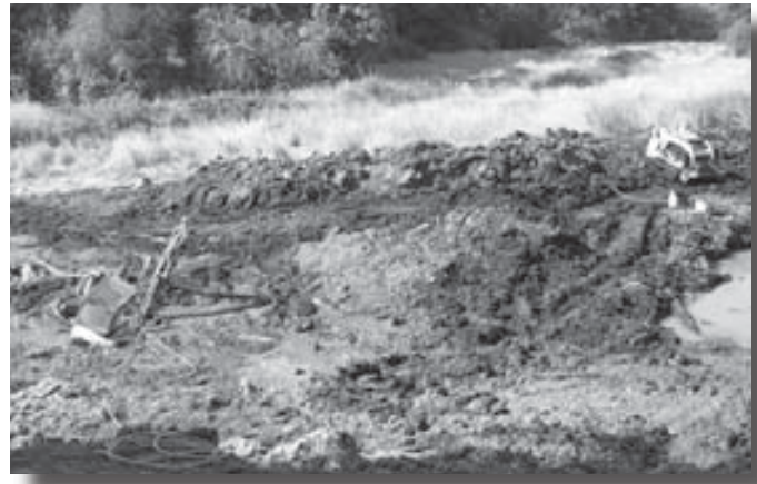
The scene at Cam's property in Gervais included an excavator buried up to its cab (left). Photo by Corrie Veenstra.
