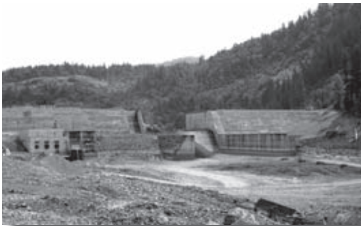
Elk Creek Dam blocked fish migration until the Corps notched the project in August 2008.
