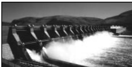
Truck and barge transport and spill for fish.
