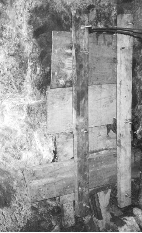
Figure A1.—Installed pressure cell.
