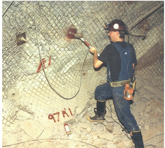
Figure 5.—Creating a source of seismic waves.
