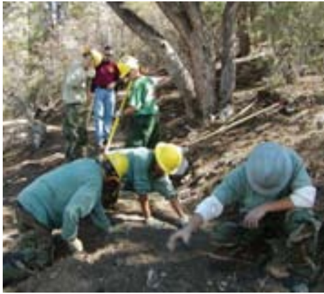
A trail maintenance crew at work
