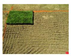
Figure 3. Install the first piece along a straight edge.
