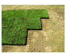
Figure 4. On each row of sod, stagger the joints as when laying bricks.
