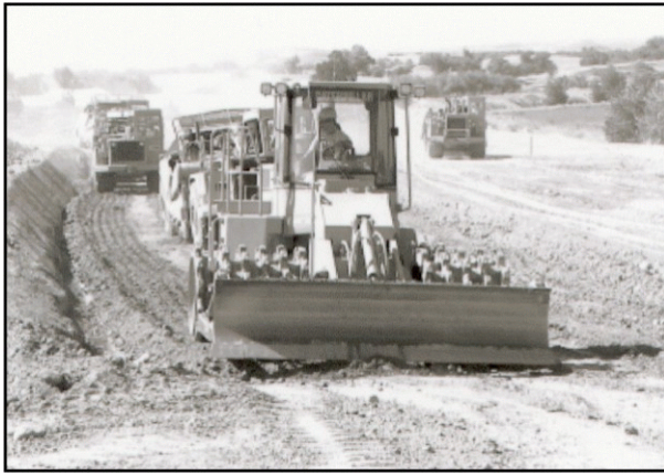
Operating construction equipment at a training site in California.
