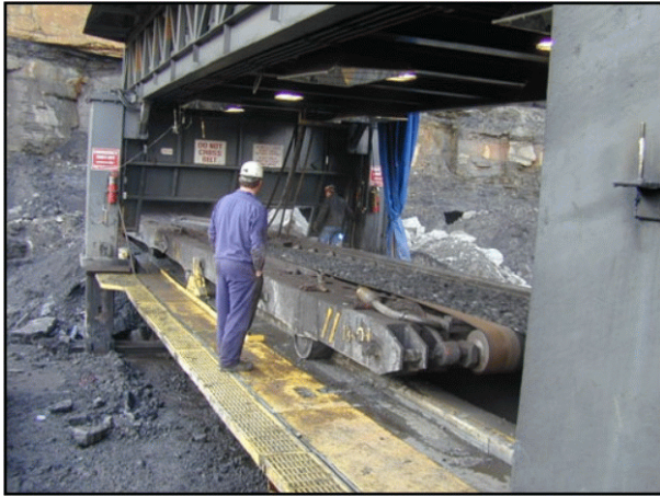
Workers around a highwall mining conveyor system.
