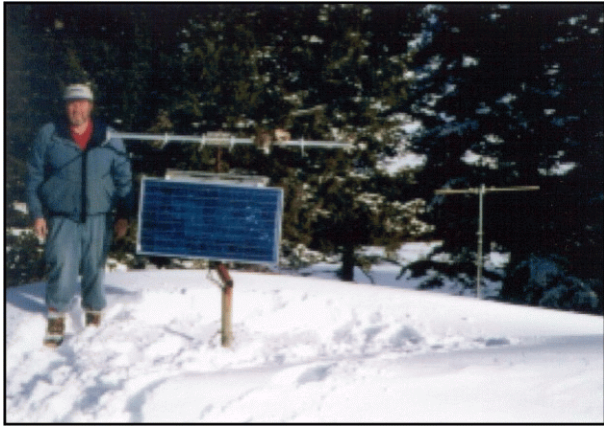
Solar-powered repeater station transmitting seismic data from the Stillwater Mine.
