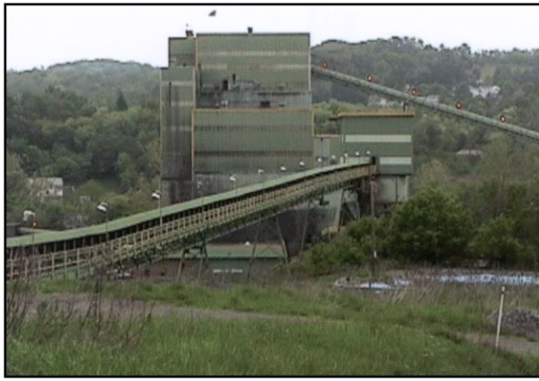
A coal prep plant.
