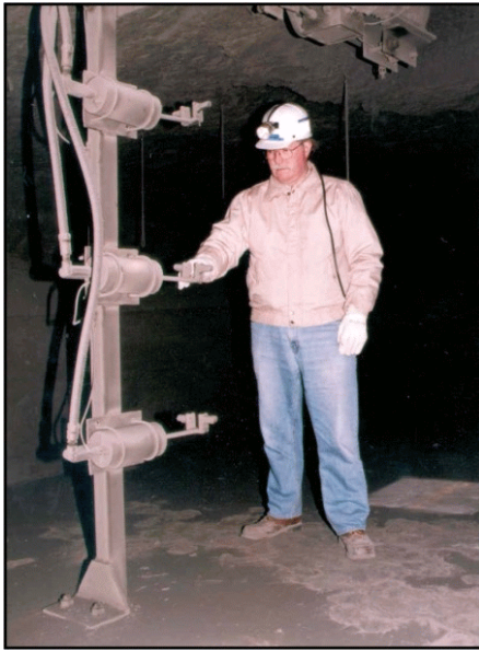
Optical dust probes used to study dust dispersion in the Lake Lynn Experimental Mine.
