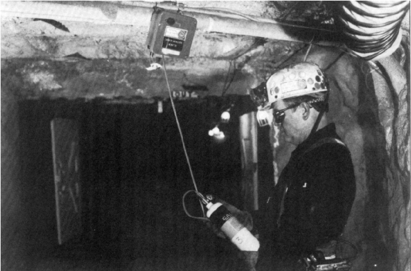
Underground test of CO remote sensing unit.
