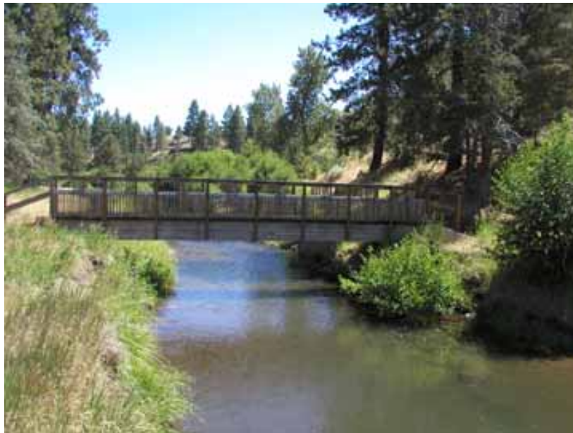
Footbridge at Sprague River Park.
