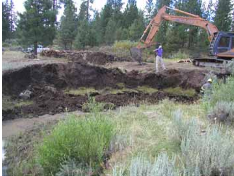
Excavator building new floodplain, then laying sedge mats.
