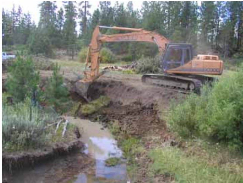
Excavator placing sedge mat on new floodplain.
