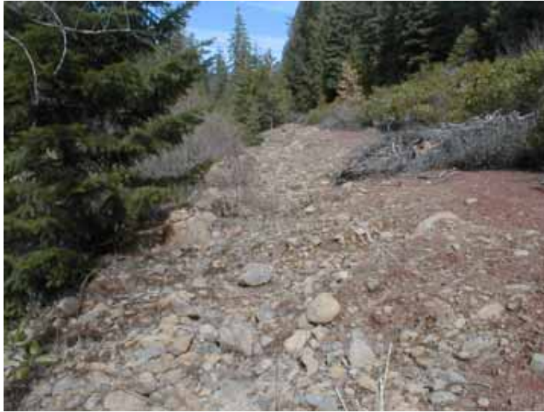
Road 060, to be decommissioned.
