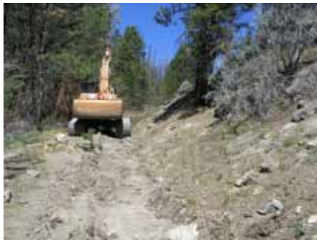
Road near channel before obliteration – initially ripped to break up compaction.
