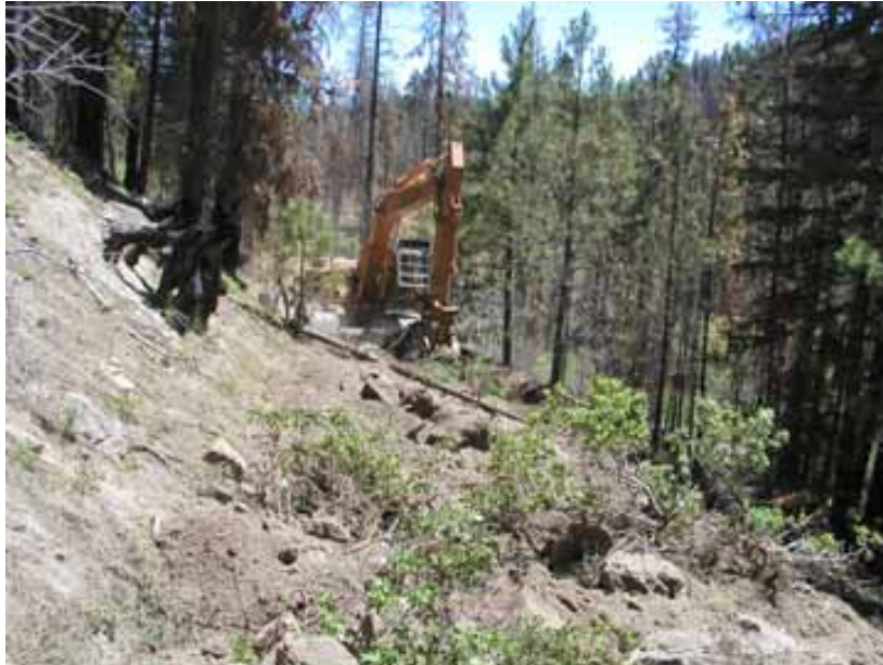
Excavator obliterating road, restoring the natural contours.
