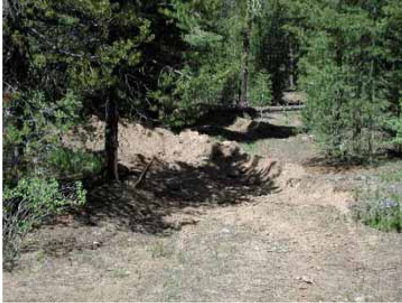
Waterbar on road that has naturally revegetated.
