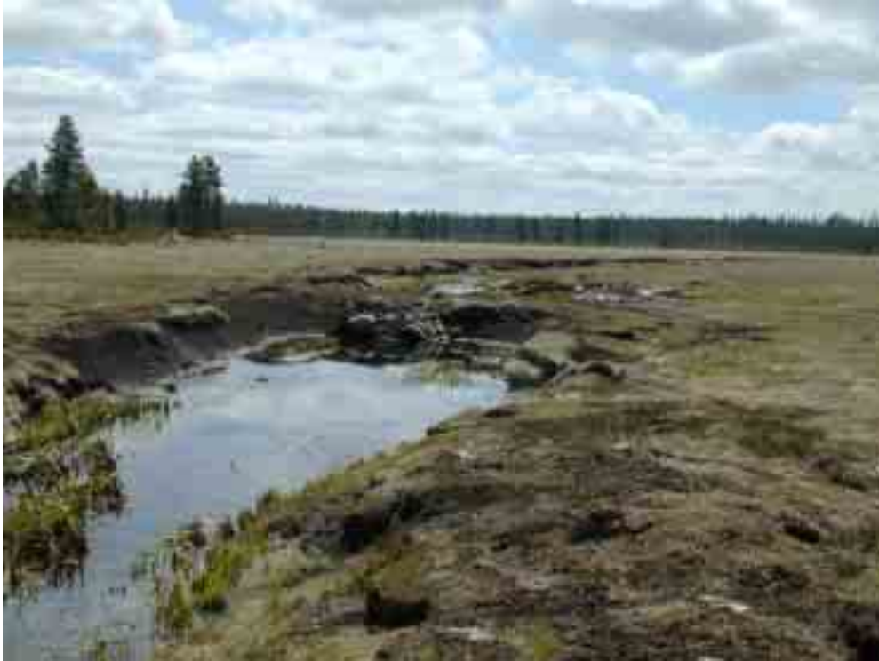
Photo 1: BEFORE photo taken at the lower end of the meadow of the main ditch where a crossing was developed for vehicle crossing.
