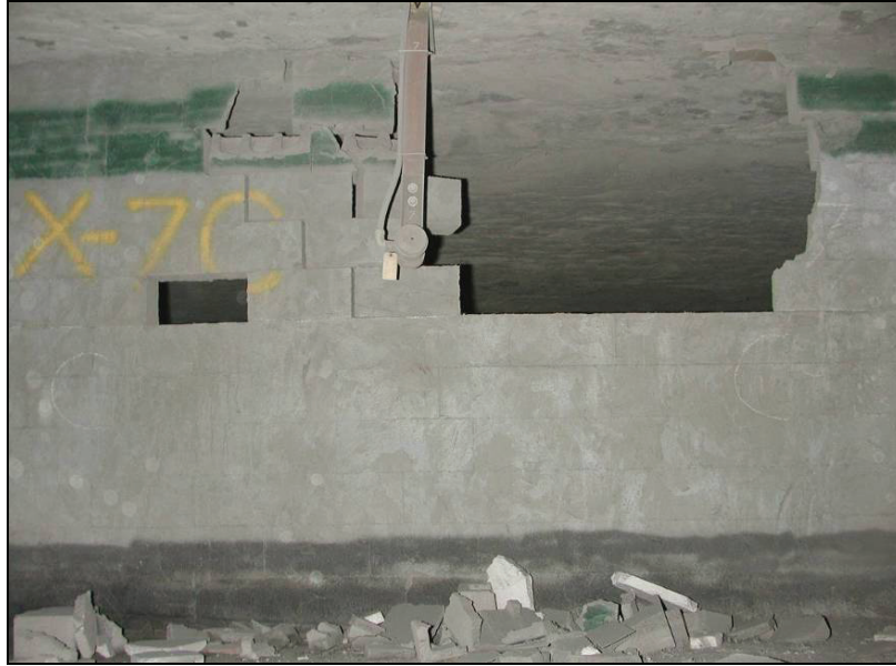
Figure 60.—Crosscut 7 dry-stacked hollow-core concrete block stopping viewed from C-drift after LLEM test #434.
