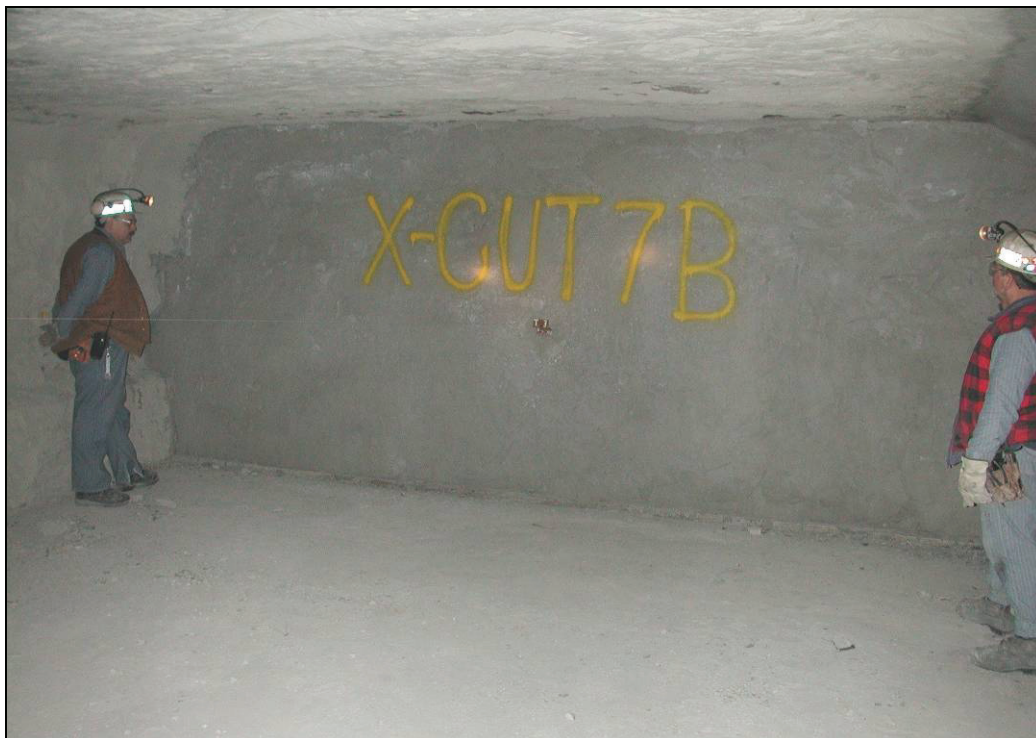
Figure 48.—The dry-stacked hollow-core concrete block stopping in X-7 remained intact after LLEM test #430.
