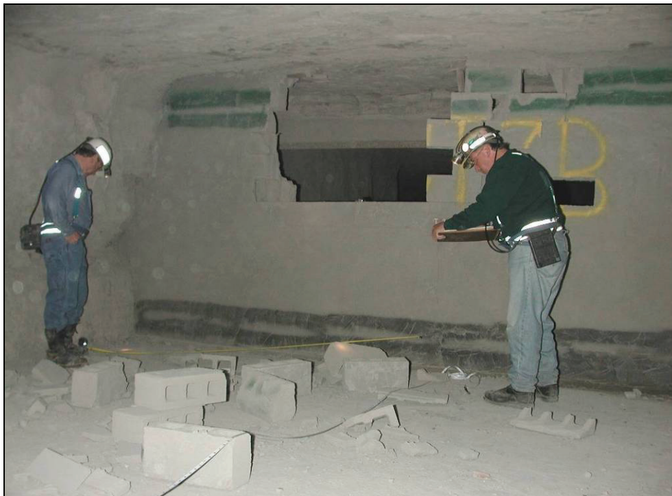
Figure 59.—Crosscut 7 dry-stacked hollow-core concrete block stopping viewed from B-drift after LLEM test #434.
