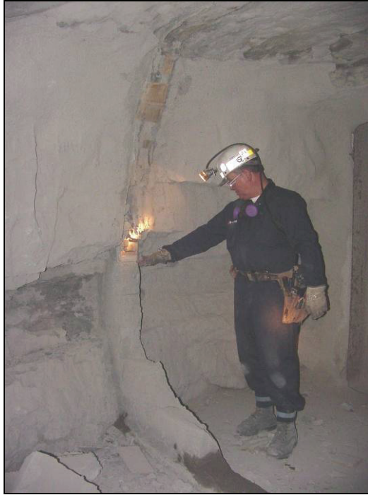
Figure 78.—Remaining blocks from the dry-stacked solid-concrete-block stopping at the inby rib in X-5 after LLEM test #463, viewed from B-drift.
