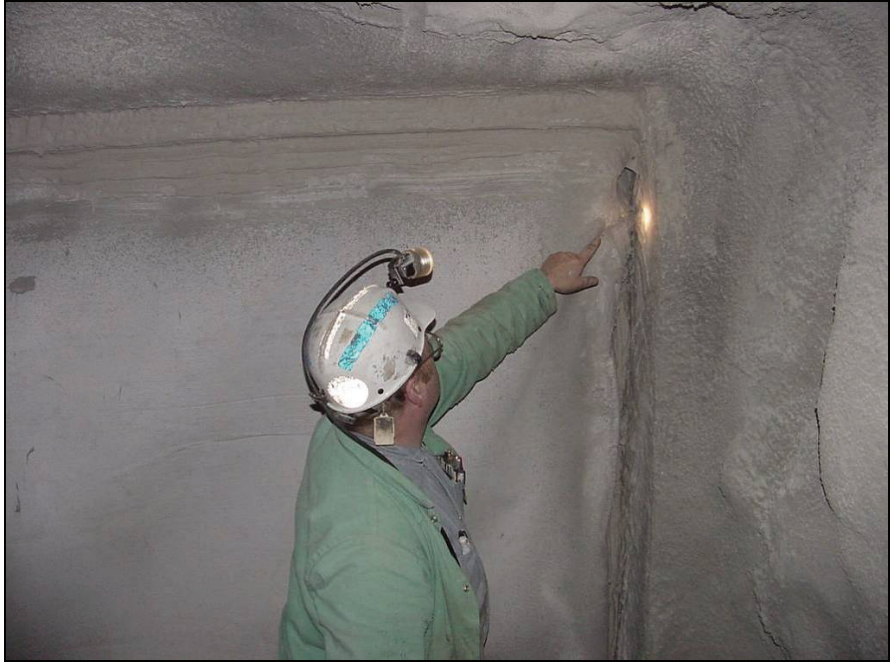
Figure 29.—Sealant along perimeter of the stopping, viewed from C-drift.
