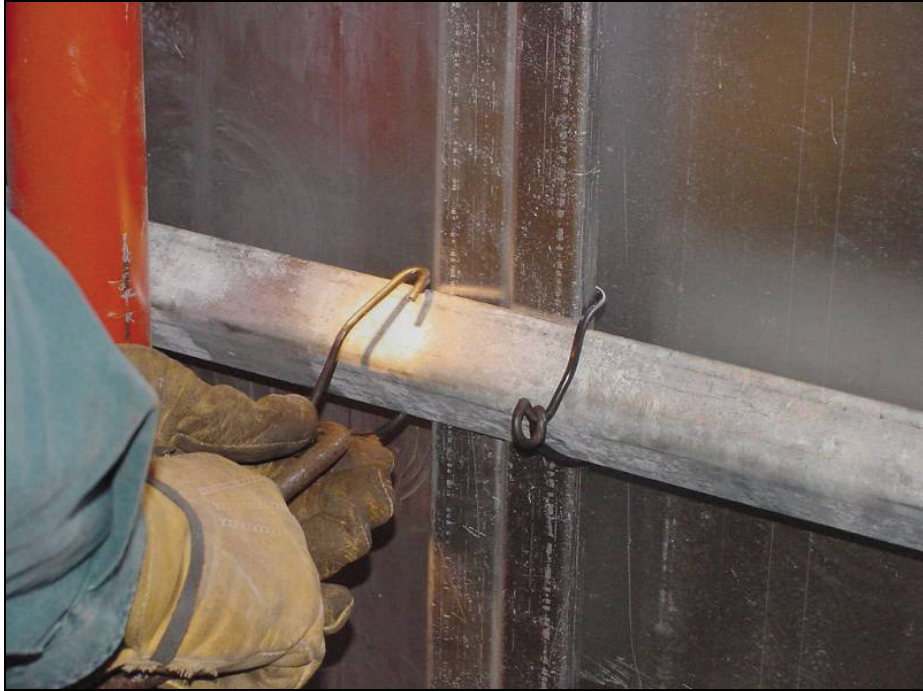
Figure 19.—Metal twist clamp used to secure open side of panel to the horizontal angle.
