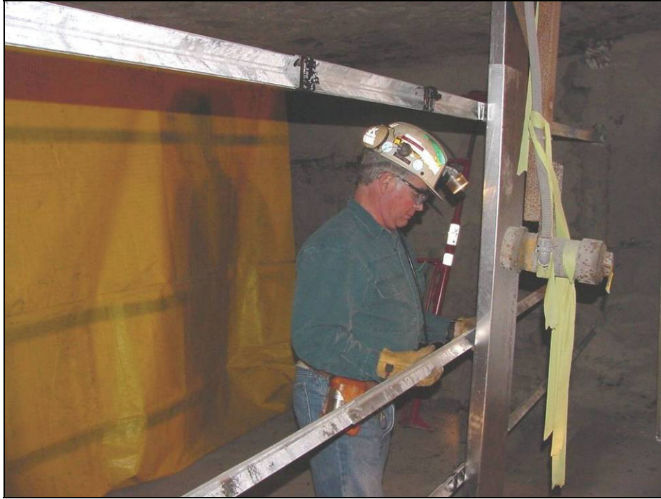
Figure 14.—Horizontal steel angles for attaching the steel stopping panels. The photo also shows the installed center panel.
