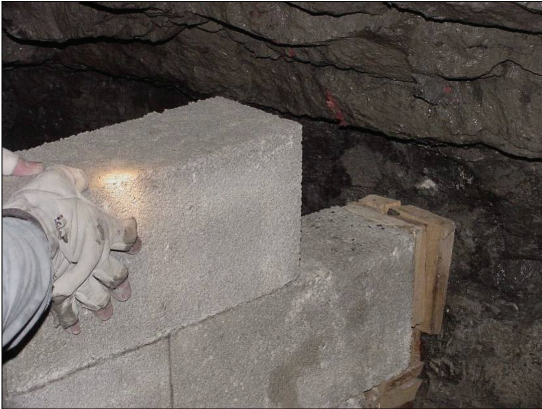
Figure 8.—Dry-stacked solid-concrete-block stopping construction with staggered joints.
