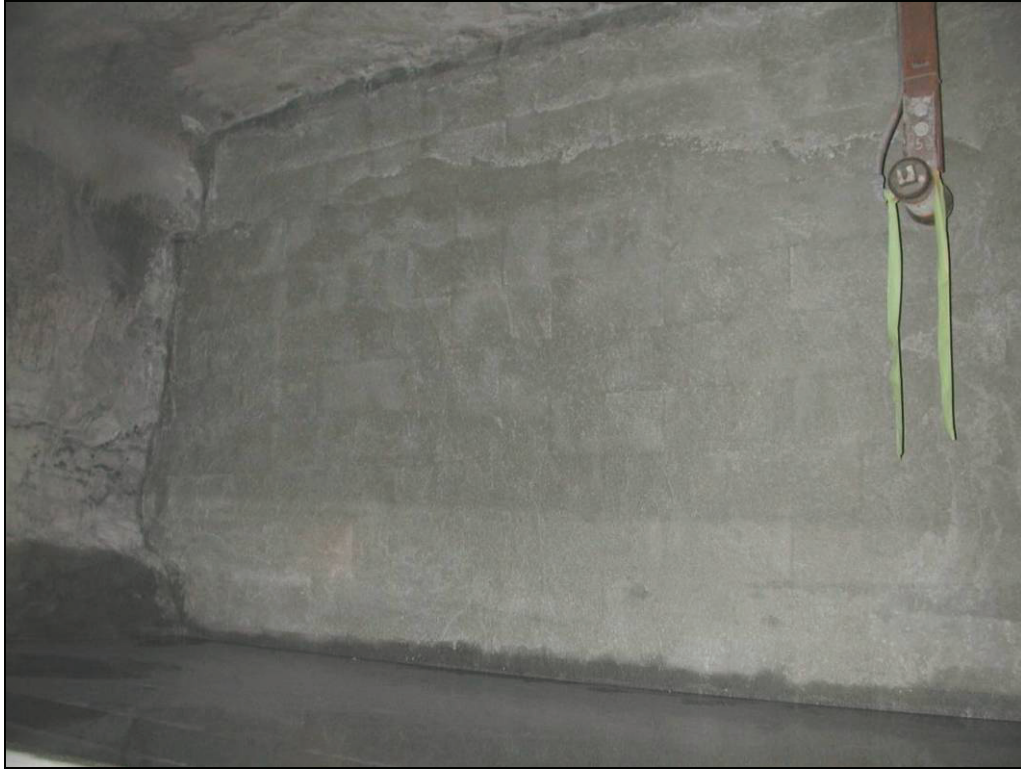
Figure 11.—Completed dry-stacked solid-concrete-block stopping in X-5 as viewed from C-drift, with the total explosion pressure transducer at the upper right.
