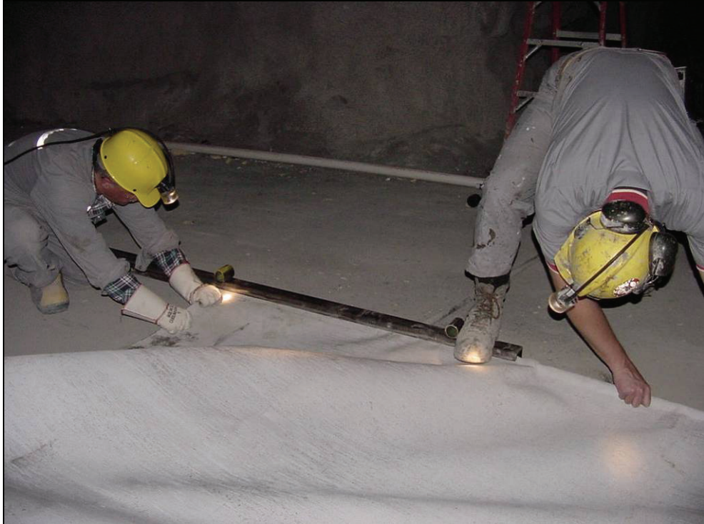
Figure 26.—Inserting pipe/sleeve into top box section.
