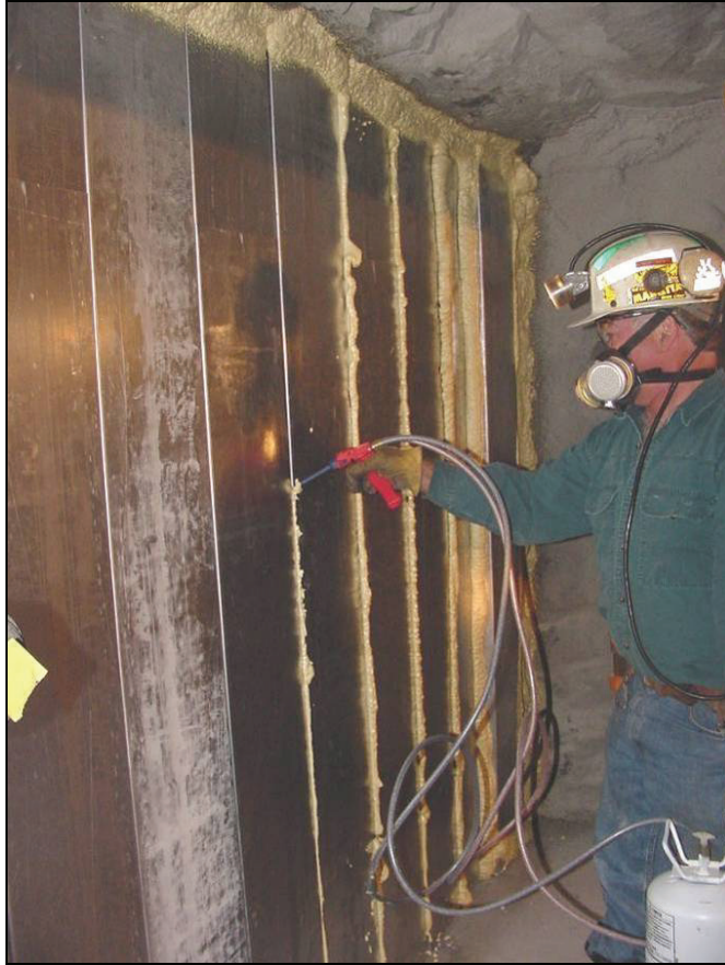
Figure 22.—Polyurethane sealant used on perimeter and vertical panel joints.
