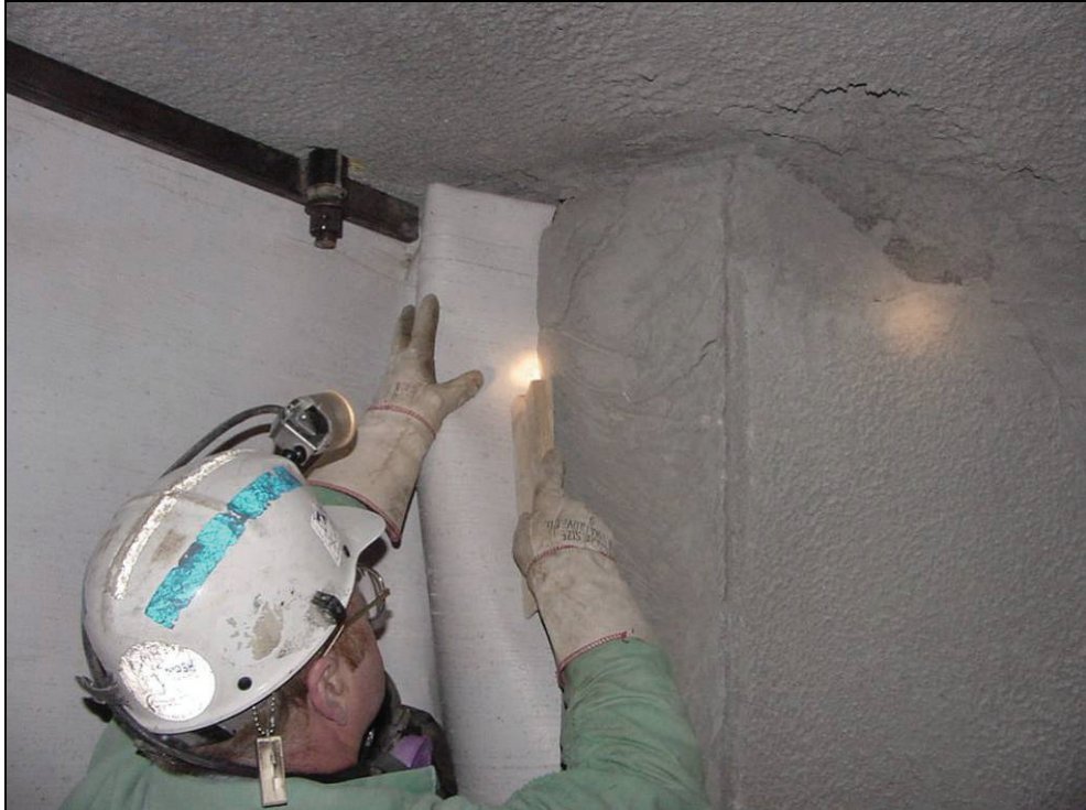
Figure 28.—Wedging woven cloth into mine rib.
