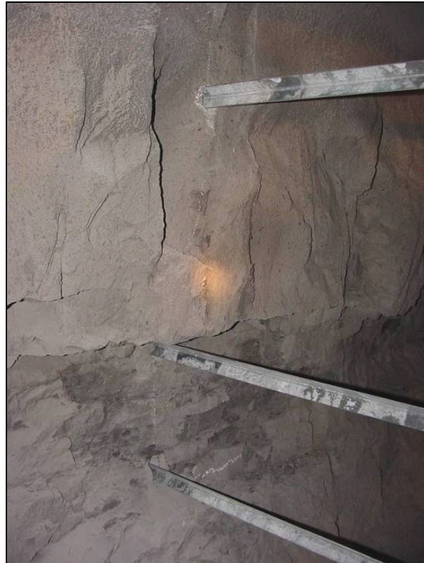
Figure 15.—Three horizontal steel angles inset into rib.
