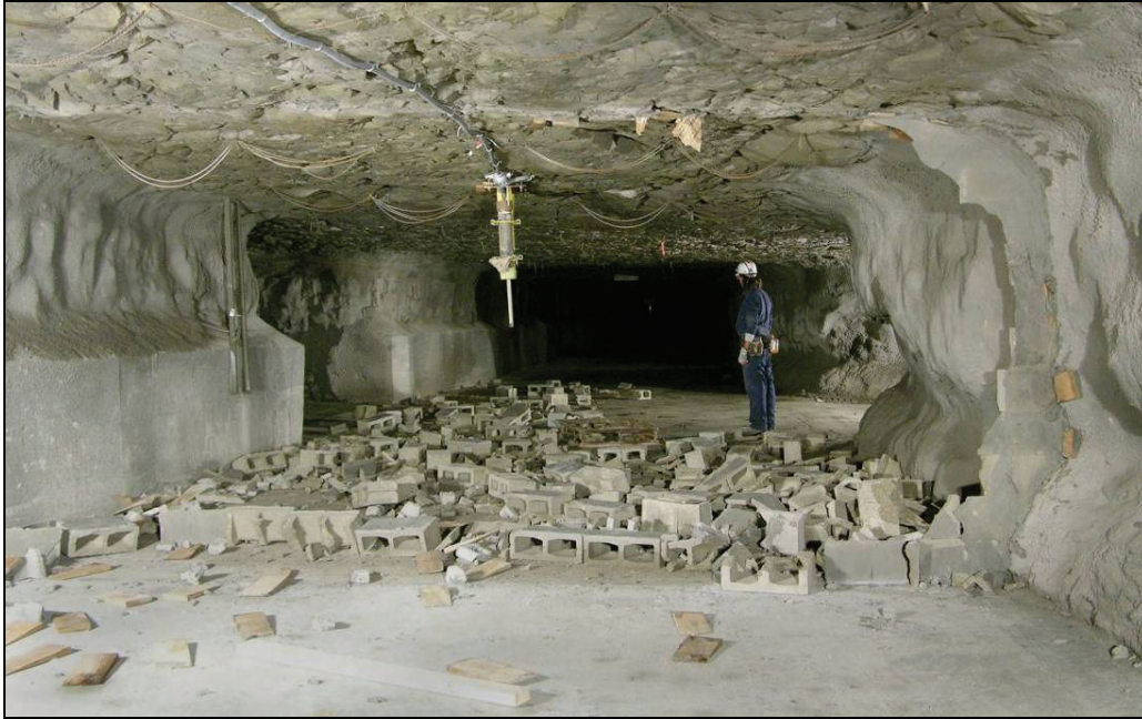
Figure 89.—Debris from the dry-stacked hollow-core concrete block stopping across B-drift after LLEM test #497.
