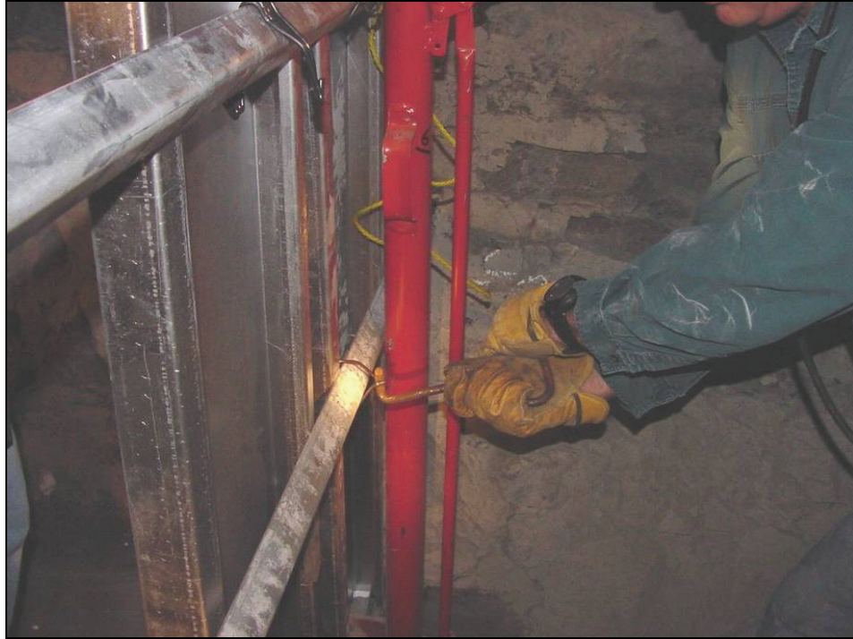
Figure 16.—Horizontal steel angles (with open sides facing panels on left), as viewed from B-drift.
