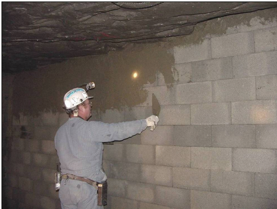
Figure 7.—Coating the dry-stacked hollow-core concrete block stopping with sealant.
