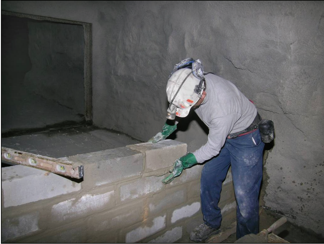
Figure 12.—Wet-laid solid-concrete-block stopping construction with staggered joints.
