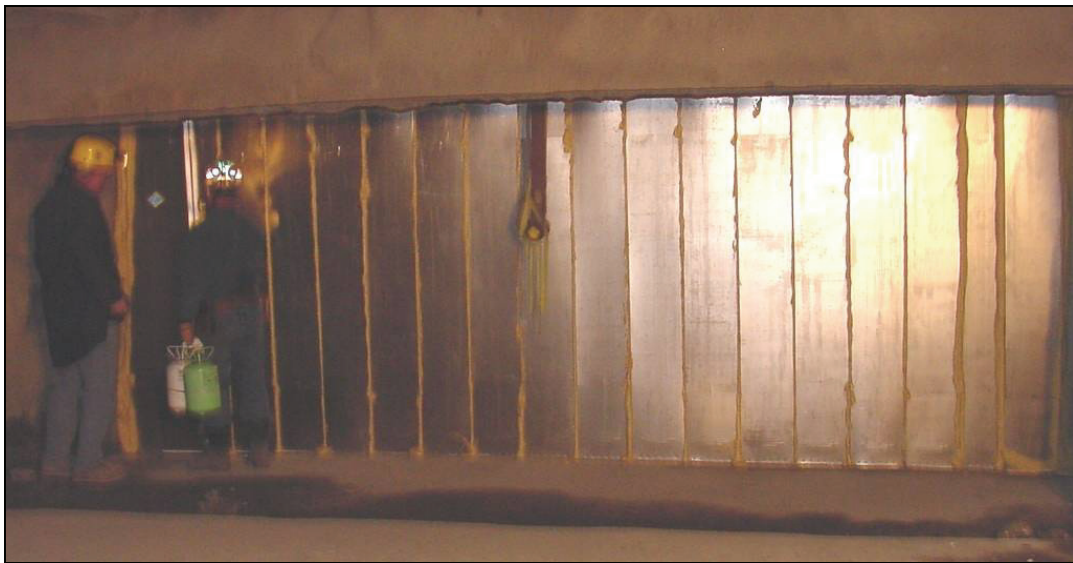
Figure 23.—Nearly completed steel panel stopping in X-6 showing closed, smooth panel sides facing C-drift.
