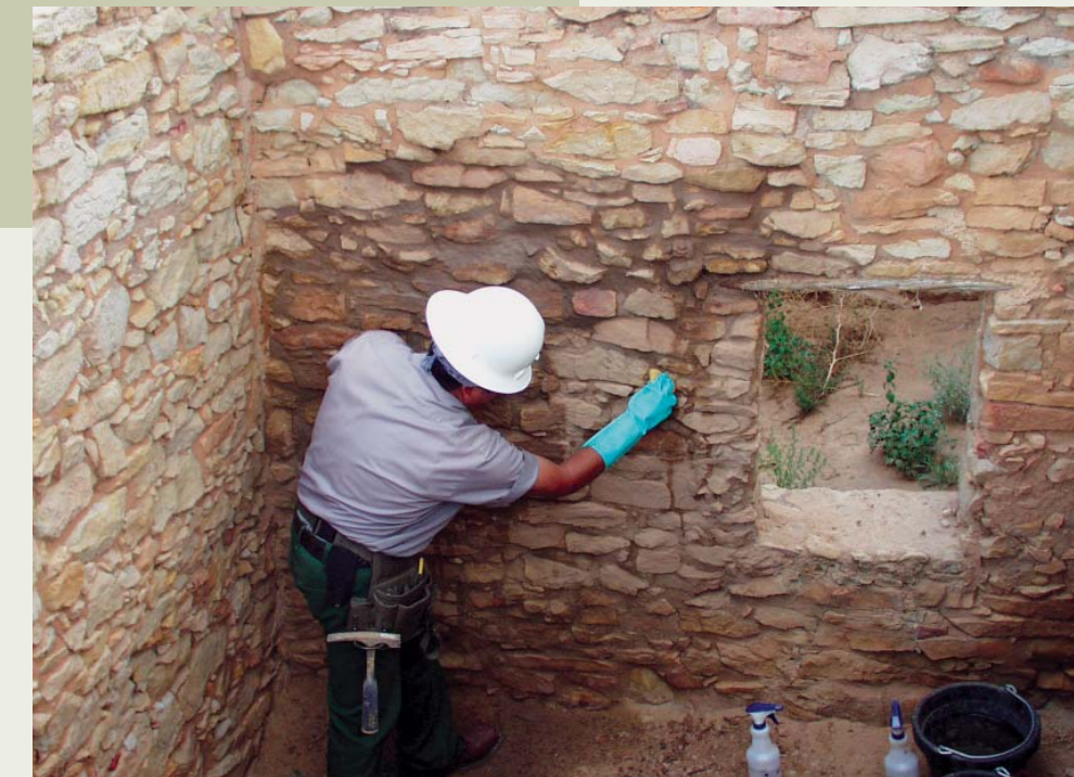
Vanishing Treasures masonry worker treating a gap in a 700-year-old wall at Atsinna Pueblo, El Morro National Monument, New Mexico. (National Park Service)
