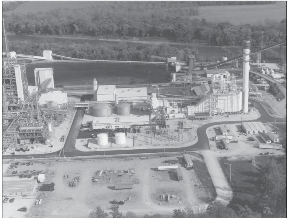
Wabash River Generating Station IGCC.
