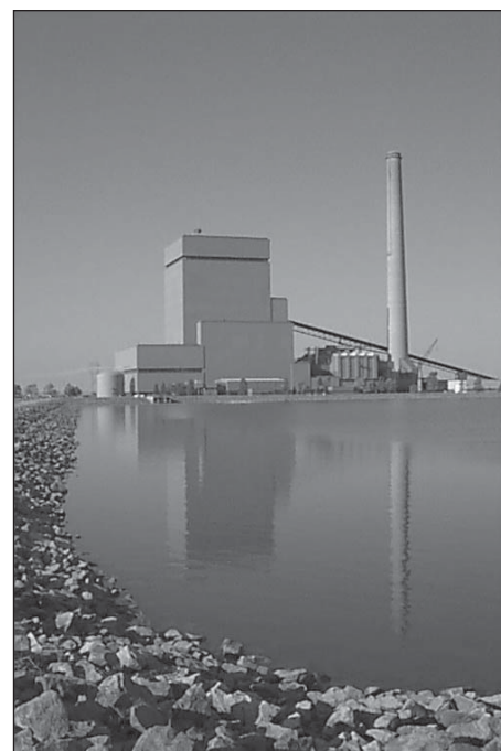
An advanced hybrid particulate collector is being demonstrated at Otter Tail Power Company's Big Stone Power Plant in Big Stone City, South Dakota.
