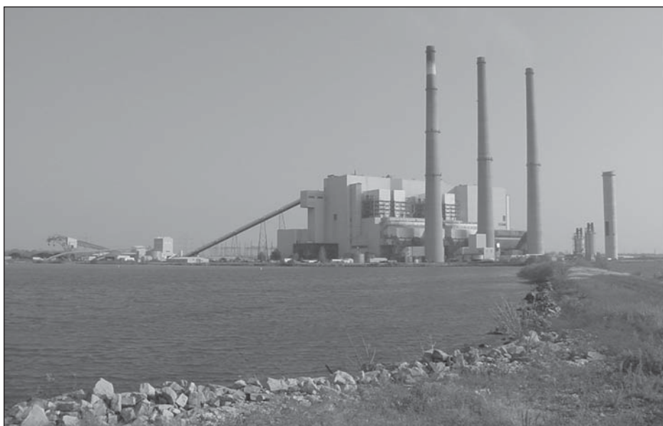
Advanced optimization software for enhanced emissions control is being demonstrated at Dynegy Midwest Generation's Baldwin Energy Complex in Baldwin, Illinois.
