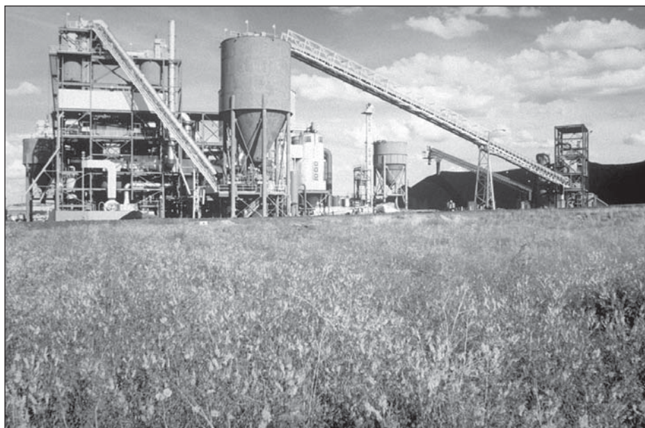
Coal feed system to ACCP to produce SynCoal®.
