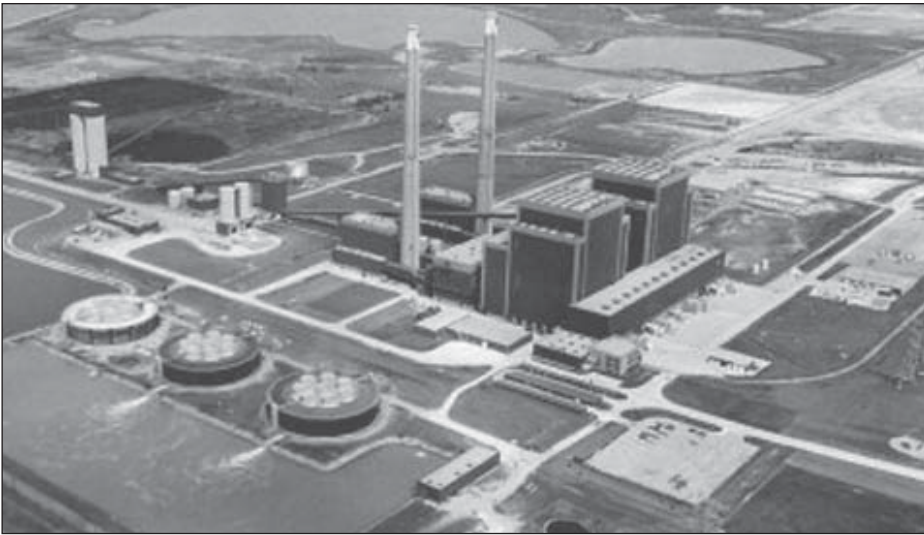
Lignite fuel upgrading is being demonstrated at Great River Energy's Coal Creek Station in Underwood, North Dakota.
