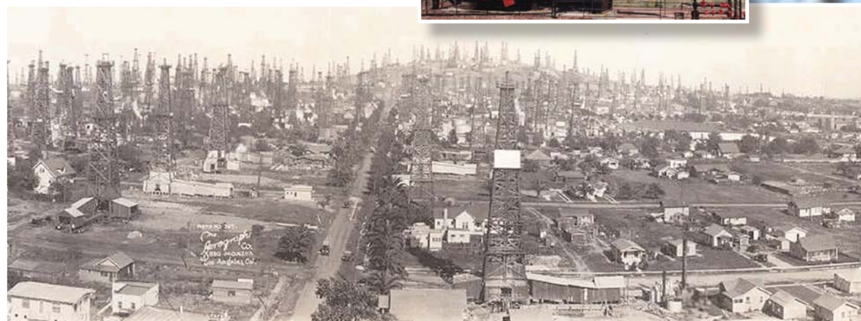
This historical photograph of Signal Hill in Long Beach, California, dates from 1923, when wells were drilled on townlots. At that time, approximately 41,000 m 3 (260,000 barrels) of crude oil was produced daily from about 300 wells, making Signal Hill the most productive field per acre worldwide, and making California the nation's top oil-producing state. Signal Hill may take on new historical significance in the 21st century as a site for geologic CO 2 storage.
