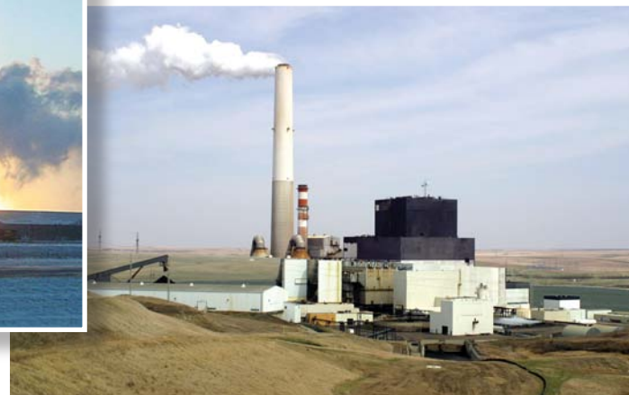
Coal-fired generation plant in North Dakota.
