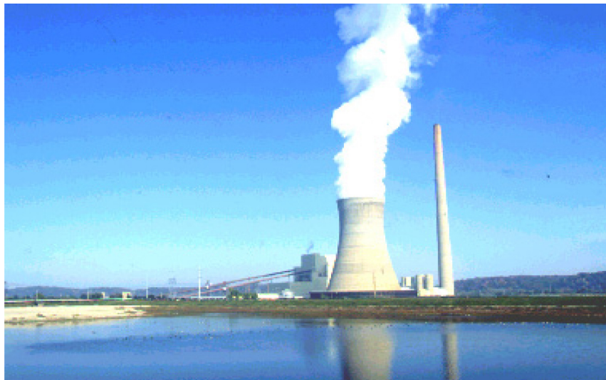
AEP's Mountaineer Power Plant in New Haven, West Virginia
