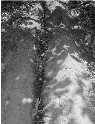
a. Trench at 1.5 m from trunk
