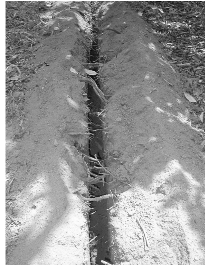
b. Trench at 2.0 m from trunk
