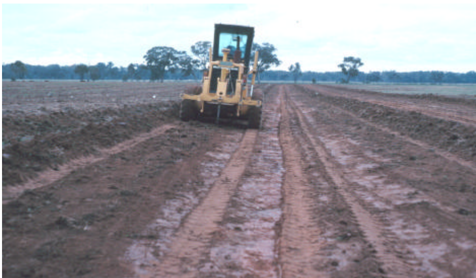
A road grader hills the soil to create a treeline bank
