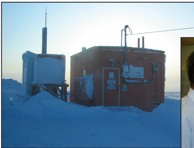
Figure 3. Well housing and methanol tank (methanol injection is used to mitigate hydrate formation in the production string) at the East Barrow No. 14 well.
