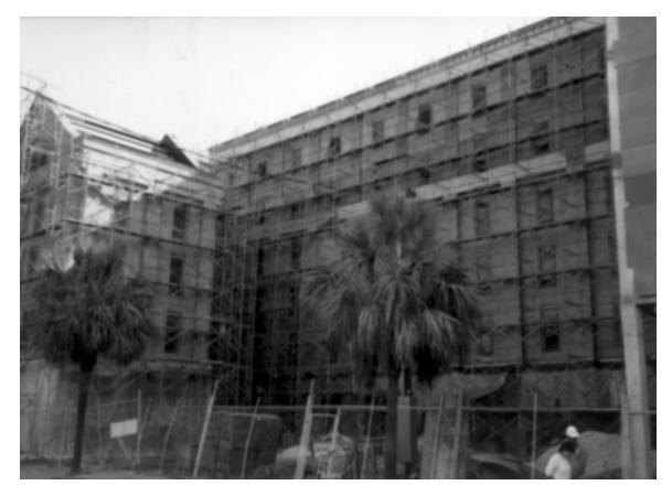
**Figure.** The victim fell from the fifth-floor level of the scaffolding shown here, when he either stood on or fell against the guardrail causing it to give way. The victim was not wearing any fall protection equipment.
