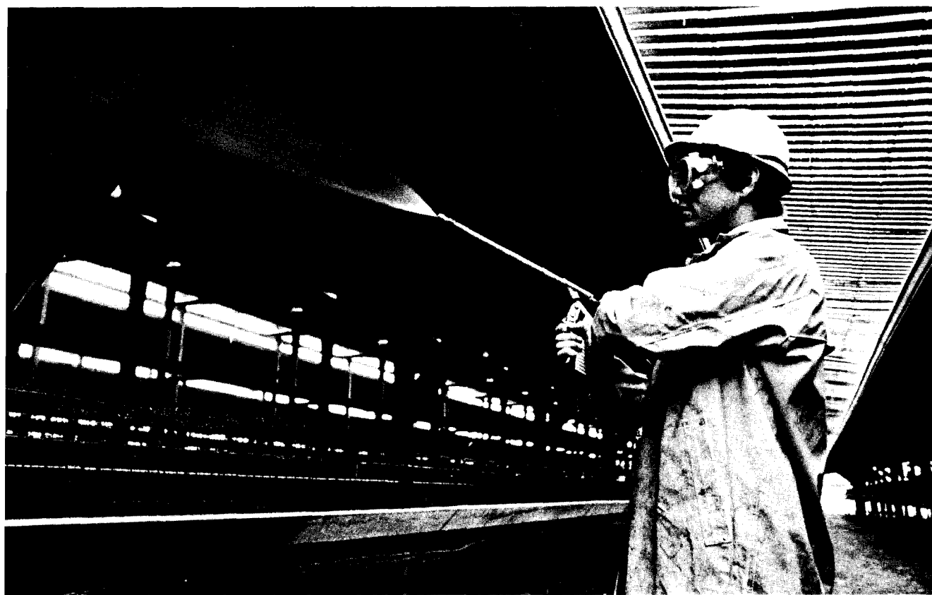
Figure 5. It is time to apply disinfectant after the building is thoroughly cleaned. Note that the worker is wearing protective gear.
