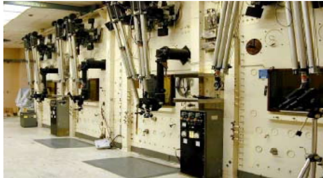
The Los Alamos Chemistry and Metallurgical Research Facility Wing 9 hot cells are used for irradiated fuel and materials examination, metallurgical examination, and neutron radiography.
