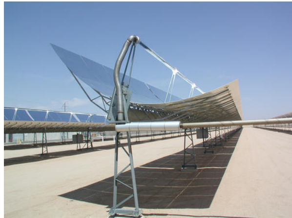
Parabolic Trough Solar Generator (Credit: Henry Price)
