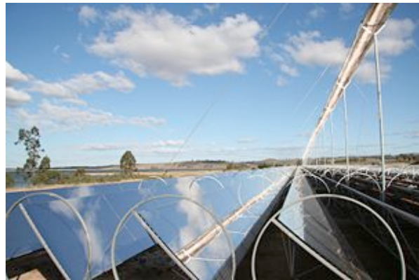
Fresnel Linear Reflector Generator (Credit: Ausra)
