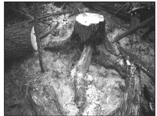
Burned and severed roots – high failure potential. Tree felled.
