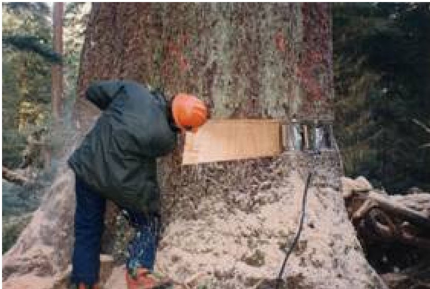
When the falling of oversized timber is taking place under extra ordinary circumstances, make sure your Fallers have proper jacks.
