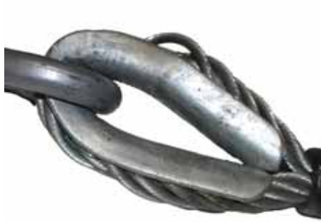
Figure 9. Deformed Thimble and Hook.
