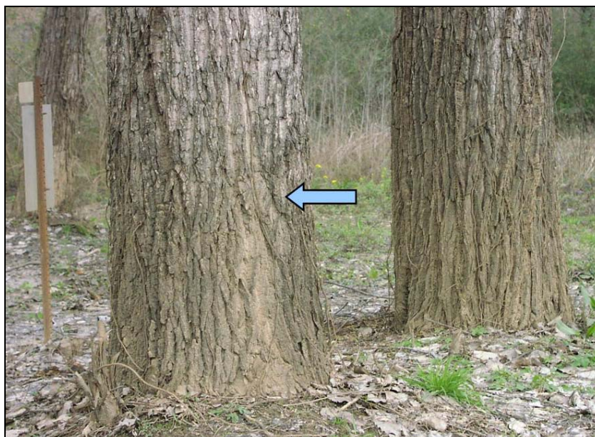
Figure 27. Silt deposit left after a recent high-water event forms a tan coating on these tree trunks (upper edge indicated by the arrow).
