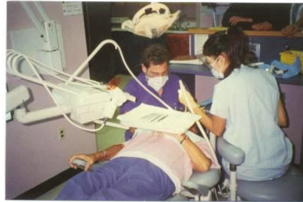
Figure 3: Over the patient dental delivery system, most commonly found in modernized or new HIS facilities.
