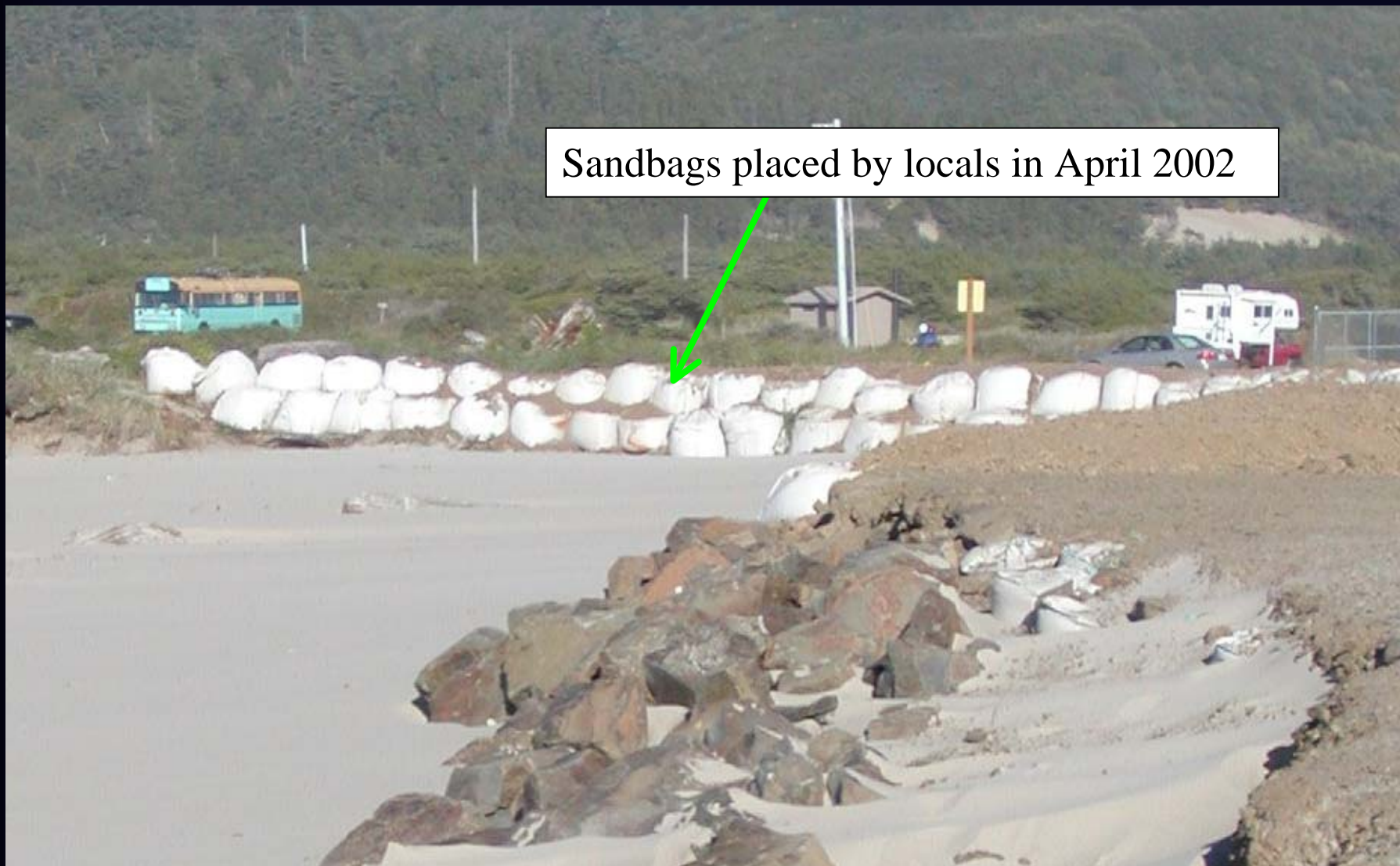
Figure 2-3 North Jetty shoreline erosion and sandbags placed in April 2002. Photo 9/23/2002
