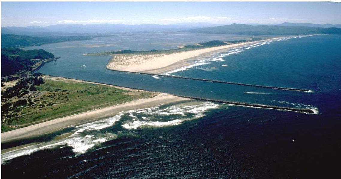
Figure 2. North and south jetties at mouth of Tillamook Bay.
