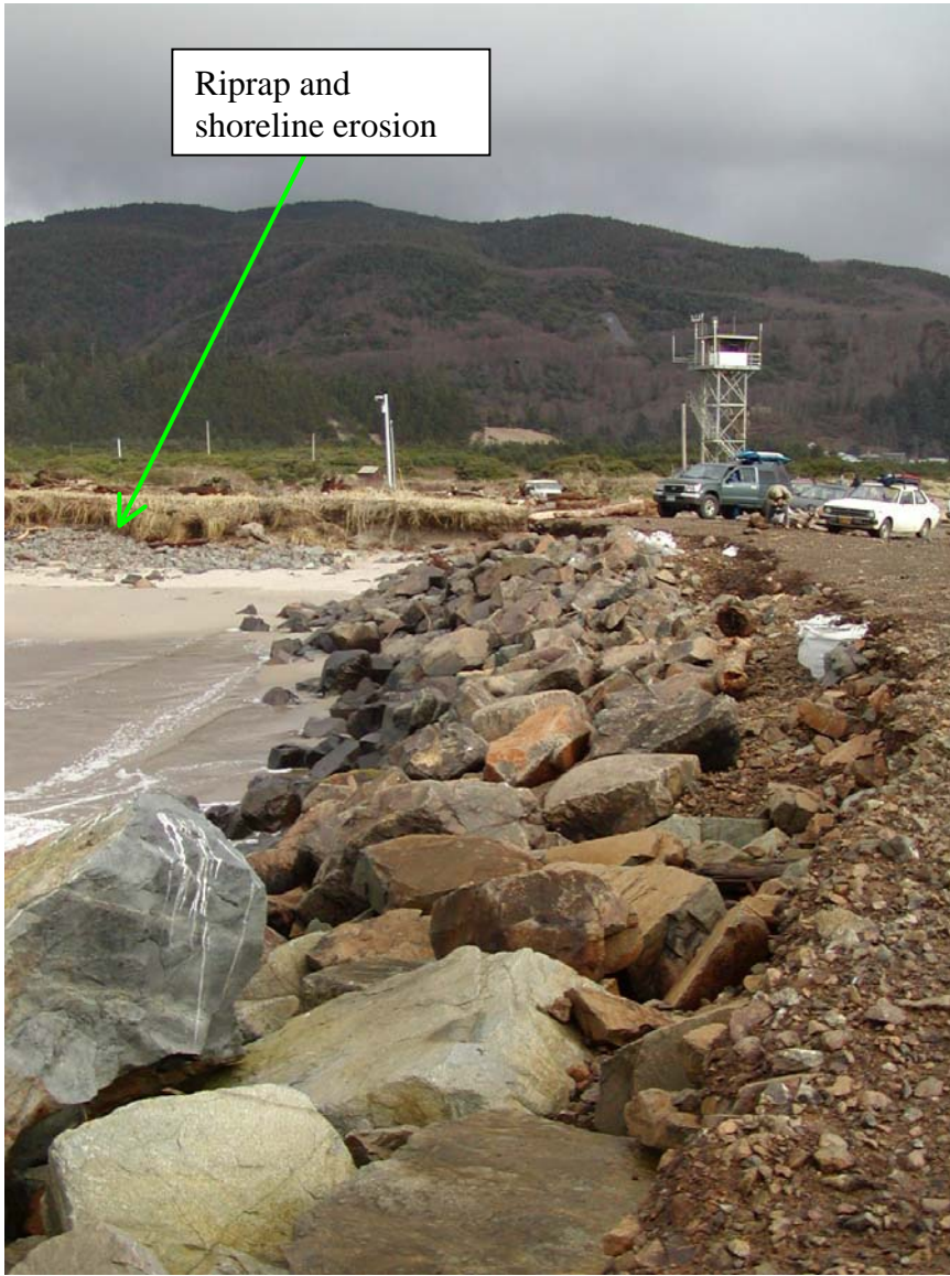
Figure 2-2 North Jetty shoreline erosion and riprap placed winter 2001. Photo 1/18/2002
