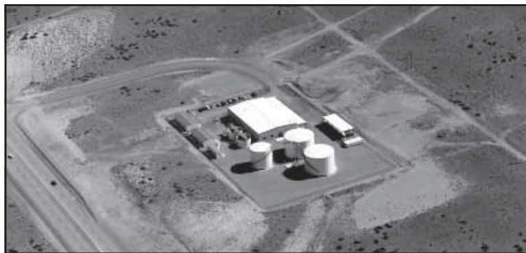
The 300 Area Treated Effluent Disposal Facility.
