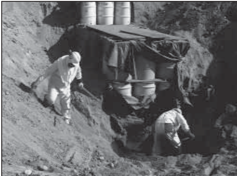
Retrieval of buried waste drums at Hanford.
