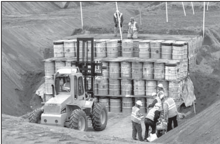
Retrieval of buried transuranic waste.
