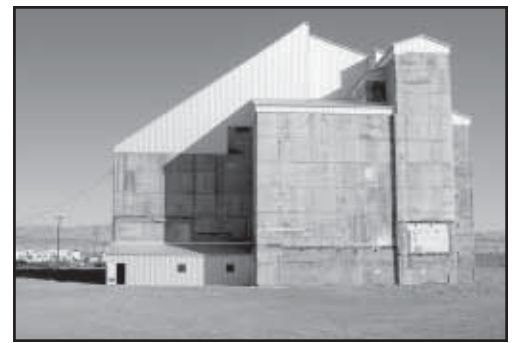
Before and after photos show the changes at DR Reactor following successful cocooning of the former plutonium reactor.
