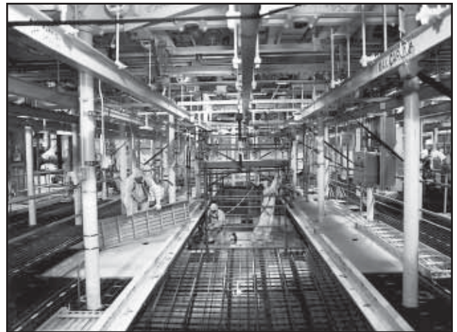
Workers at the K-West Basin.
