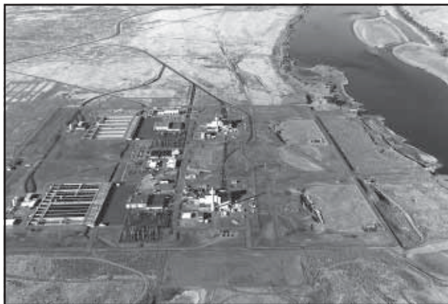
The K-Basins are located at the K-East and K-West reactors, very near the Columbia River.
