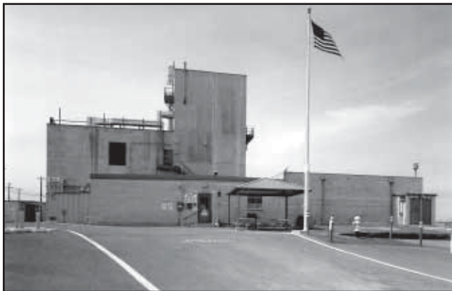
Hanford's 242-A Evaporator Facility.
