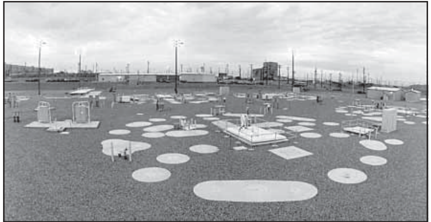
A Hanford tank farm.
