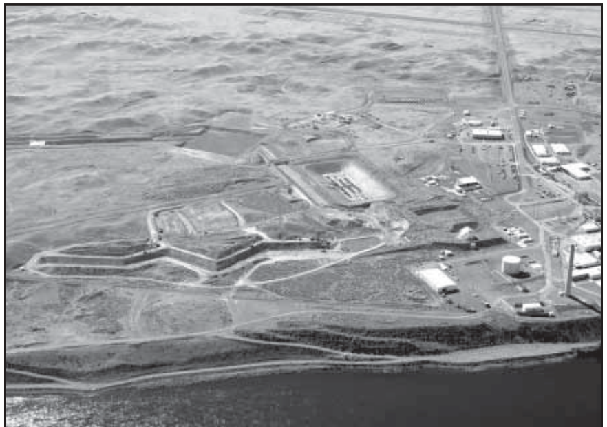
Clean-up work near the N Reactor.
