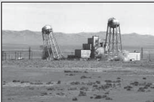
The demolition of C Reactor’s water towers.
