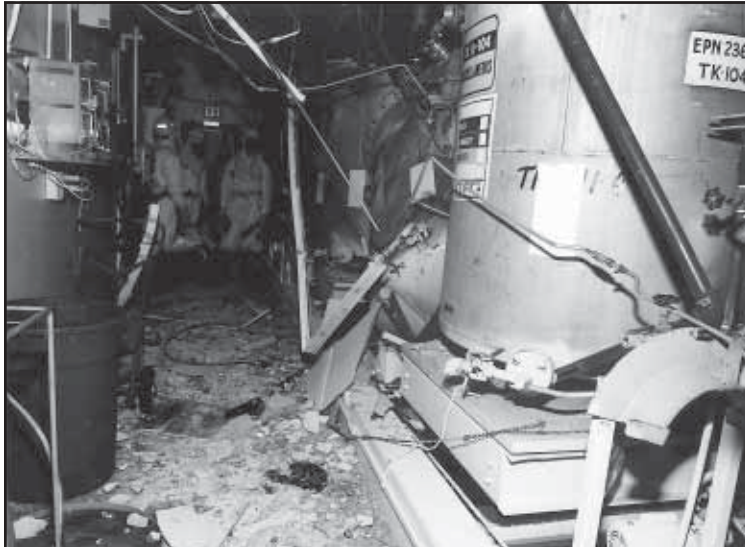
The results of a chemical tank explosion inside the Plutonium Reclamation Facility.
