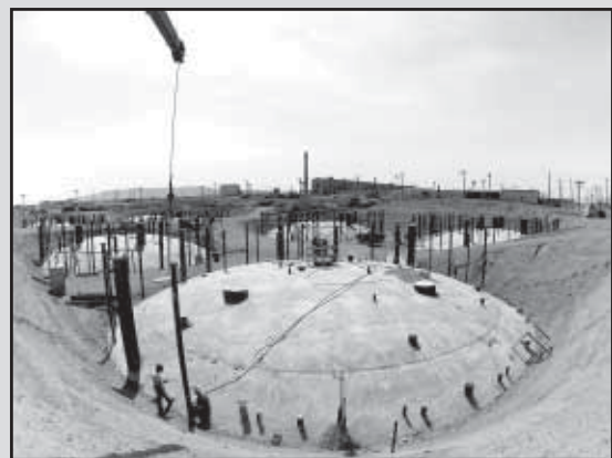
Hanford's tanks under construction.
