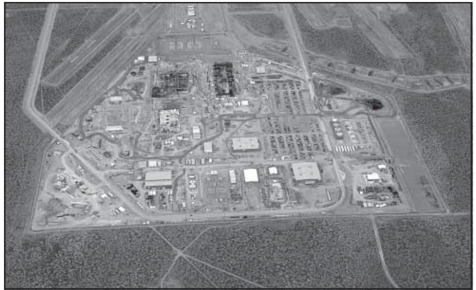
Aerial photo of the waste treatment complex in April 2004.
