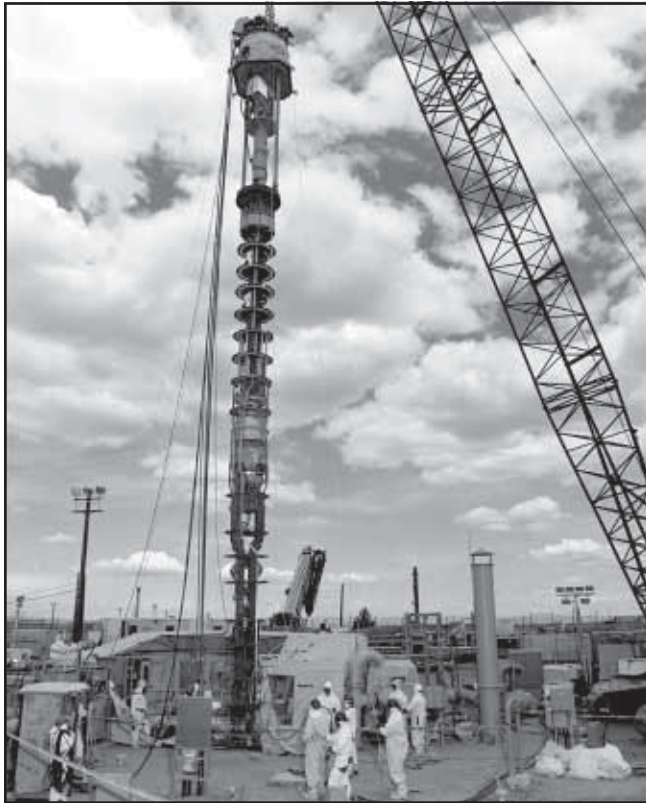
Installing the mixer pump in tank SY-101.
