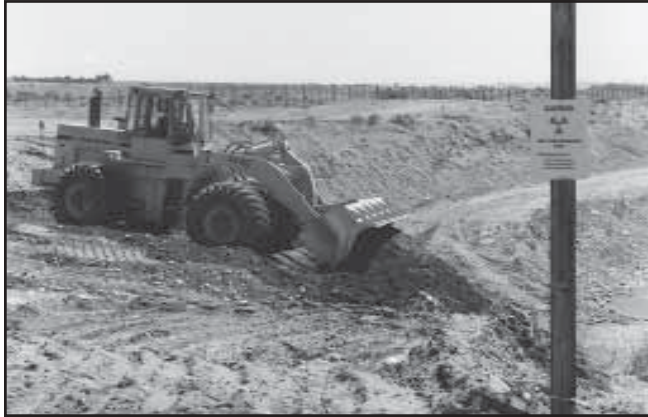
Filling waste trenches with clean dirt near Hanford's 300 Area.
