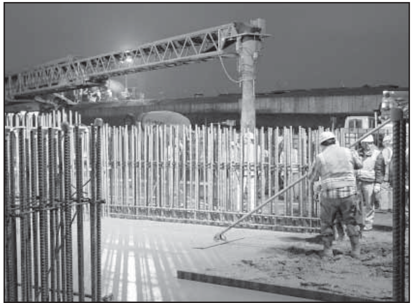
Concrete crews working in the high-level waste treatment facility.
