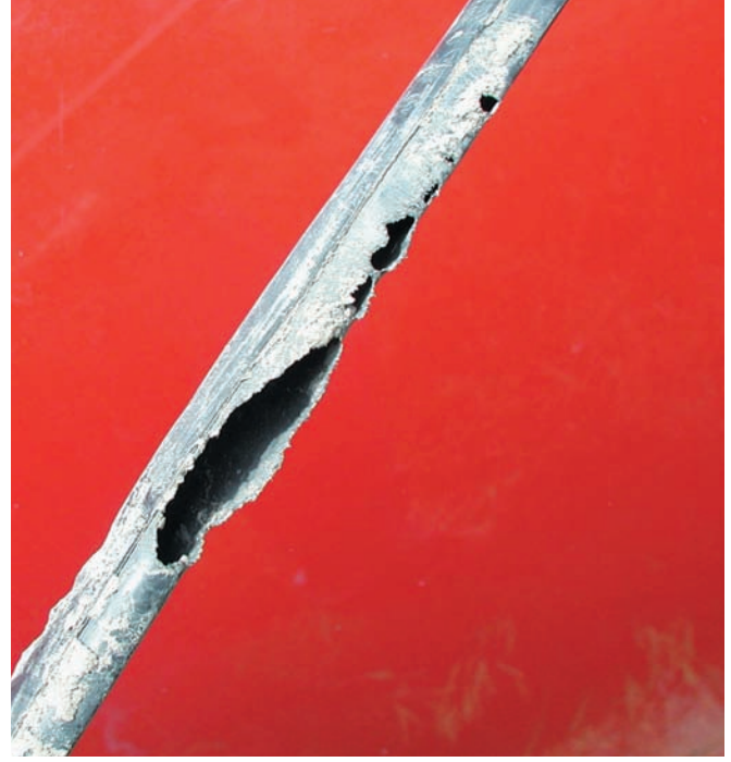
Figure 7. Damage to driplines caused by rodents.
