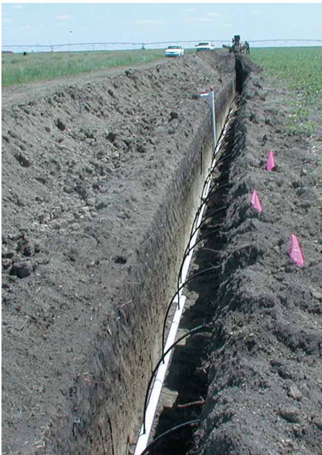
Figure 2. System installed underground.
