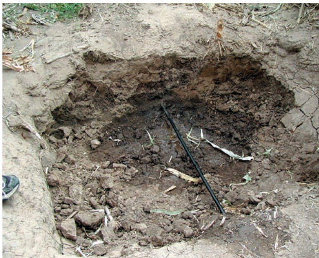
Figure 1. Dripline installed underground.
