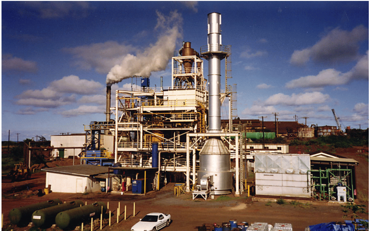
Figure 4.8: Hawaii Gasification Facility
