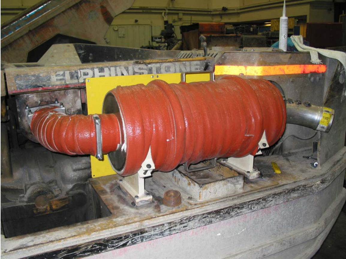
Figure 5. ECS Cattrap DPF system on the LHD #92526
