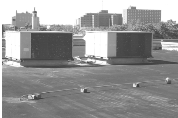
Figure 5. Back side of annex rooftop AHUs.
