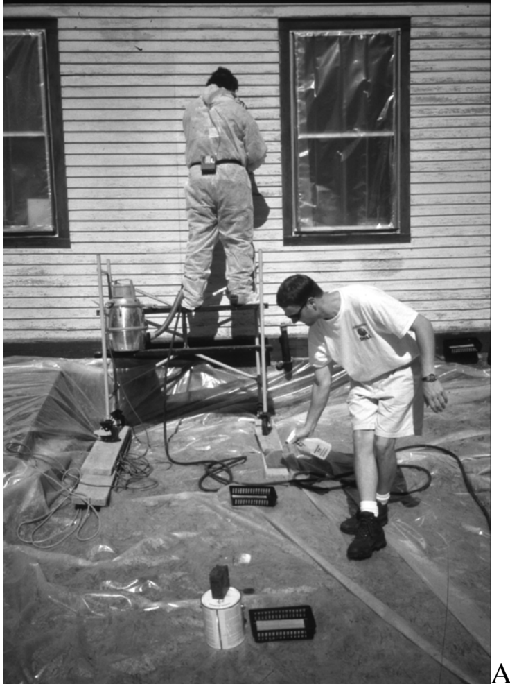
Figure 2. Sampling Set Up during a Paint Removal Method
