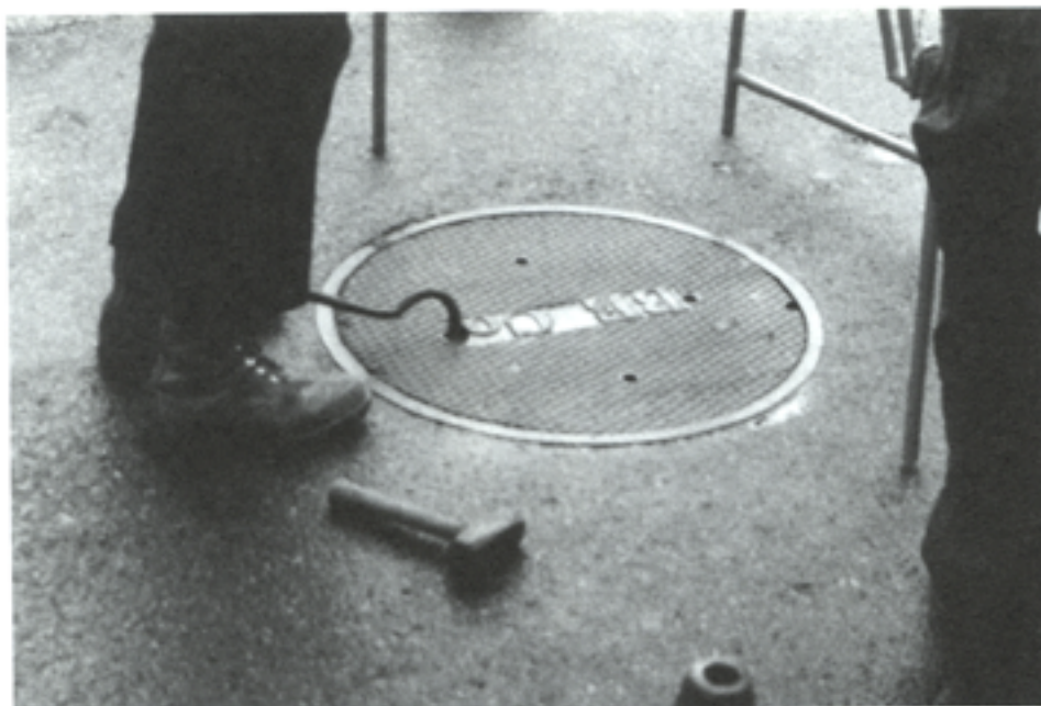
Figure 4. Use of special tool to lift UUV cover.
