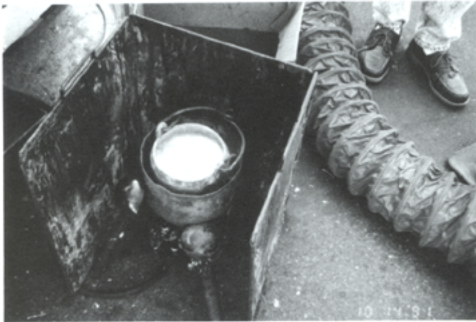
Figure 1. Lead being heated in open ladle in general vicinity of UUV.
