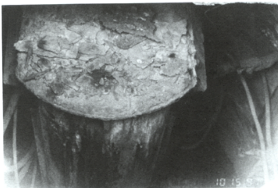
Figure 12. Photograph showing physical condition of a transformer in small UUV.
