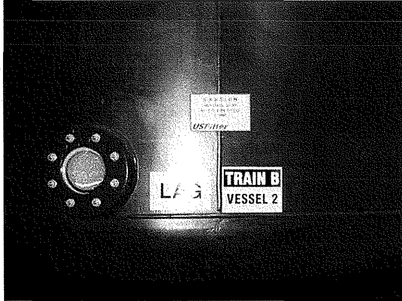
Ion Exchange Lag Vessel – Treatment Train B
