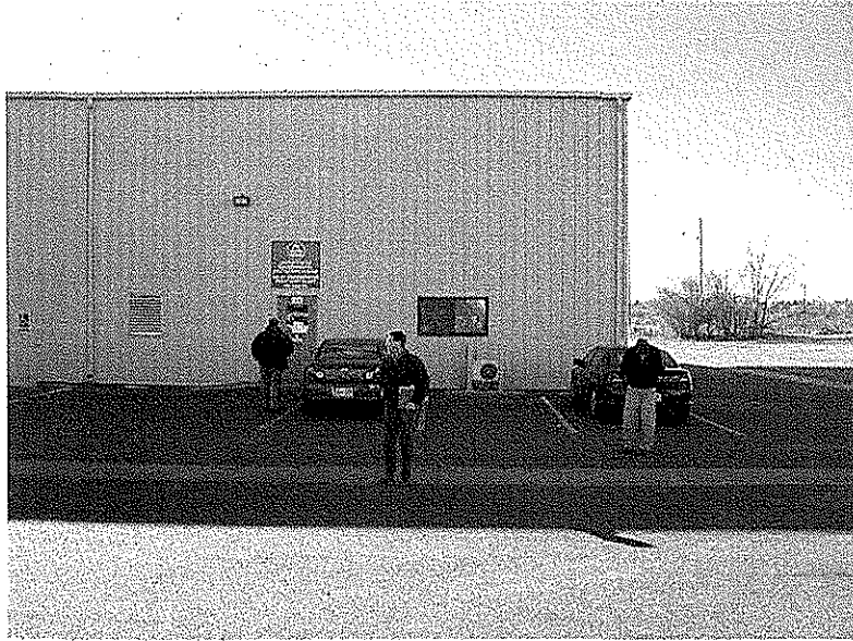
North Side of Treatment Building
