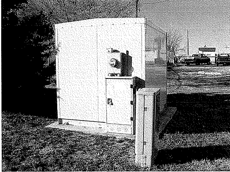
Protective Building - Former City Production Well PWS-8
