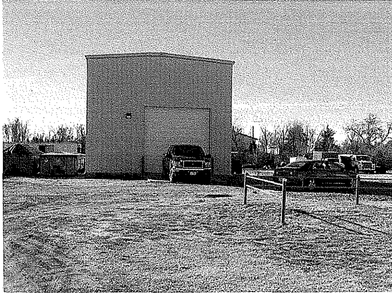
Building Housing GAC High Plain COOP GAC Unit
