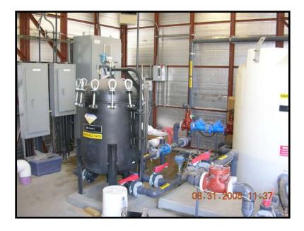
The ASTP includes pumps, filters, controllers and an air stripper unit that removes volatile contaminants from the ground water. This ground water is extracted from an extraction well, treated and re-injected into the aquifer after treatment.
