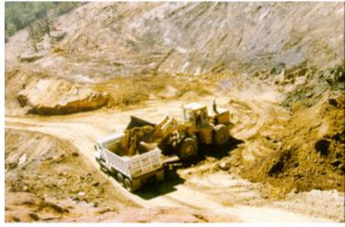
Photo #3: The tailings were taken to an on-site disposal cell where they were amended with limestone (seen in foreground) before being placed into the cell. The cell will be covered with a multi-layer cap.
