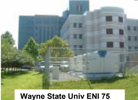
Emergency ENR2000 2MW Diesel
