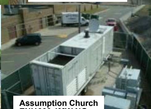
Substation Islanding ENR2000 2MW Diesel
