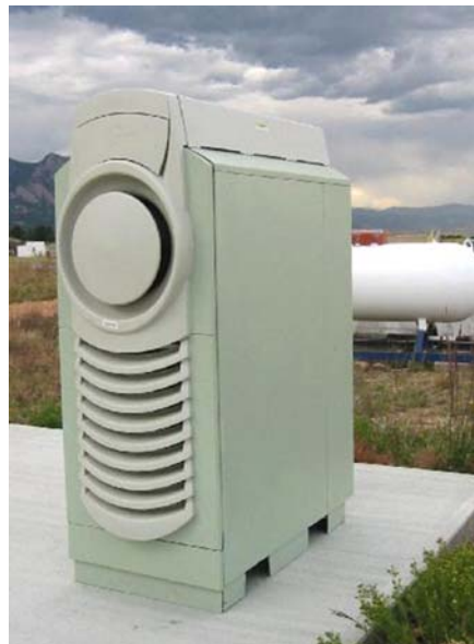
Figure 20. Microturbine (NREL 2008)
