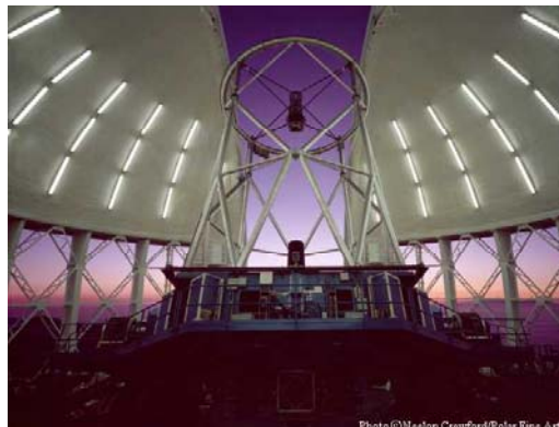
Gemini North dome/enclosure with setting sun (to left) lighting up bottom half of telescope through thermal vents (fully open). The observing slit is partially open revealing the truss and top end of the telescope. Credit: Gemini Observatory/AURA
