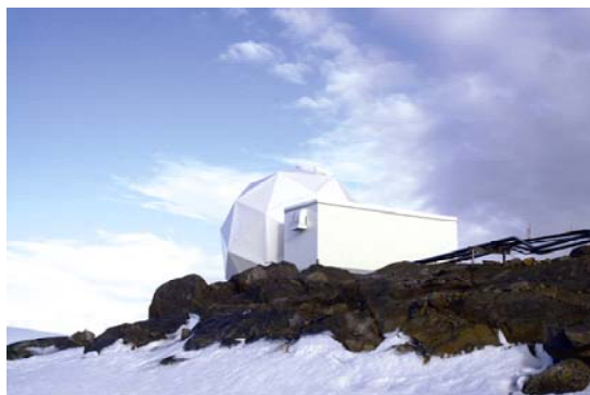
The Earth Station behind Palmer Station provides a communication link via the 5 meter diameter antenna that sees a satellite orbiting the equator, allowing people to make phone calls and use the Internet, as well as providing the remote station with telemedicine capability.
