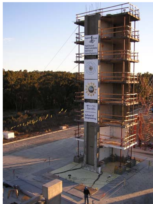
Researchers at the University of California, San Diego, in partnership with industry, use the largest outdoor shake table in the U.S. as part of NEES to test the tallest building structure ever on a shake table. This seven-story, 65-foot tall, reinforced concrete structure is being tested to investigate "promising new designs that might improve the earthquake safety of apartment and condominium buildings and other residential structures in densely populated and seismically active regions in Los Angeles and Southern California." Credit: Professor José I Restrepo, Department of Structural Engineering, University of California, San Diego
