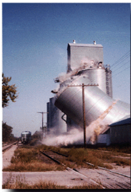
Collapse of Silo
