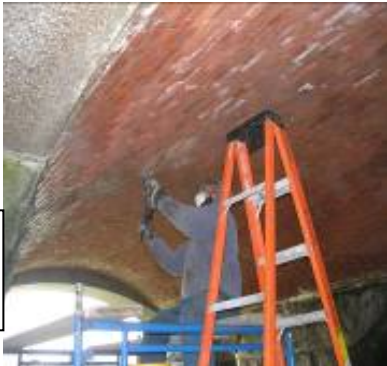
Replacing missing, broken and loose bricks at Fort Popham
