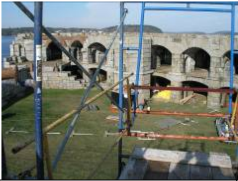
Fort Popham masonry repairs Phase 1
