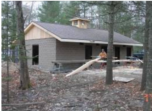
Damariscotta Lake State Park bathhouse
