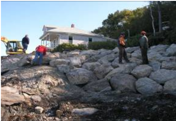
Eagle Island State Historic Site - Shoreline Erosion Protection
