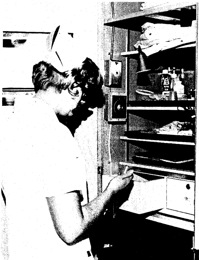
A dual-access cabinet in each room contains the patient's care plan as well as all the linens, supplies, and medications needed for his care.
